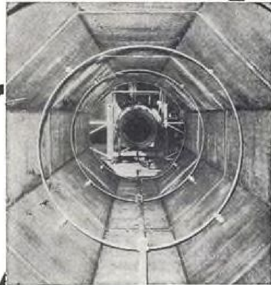
Interior of ISC Jet Aircraft Muffler
