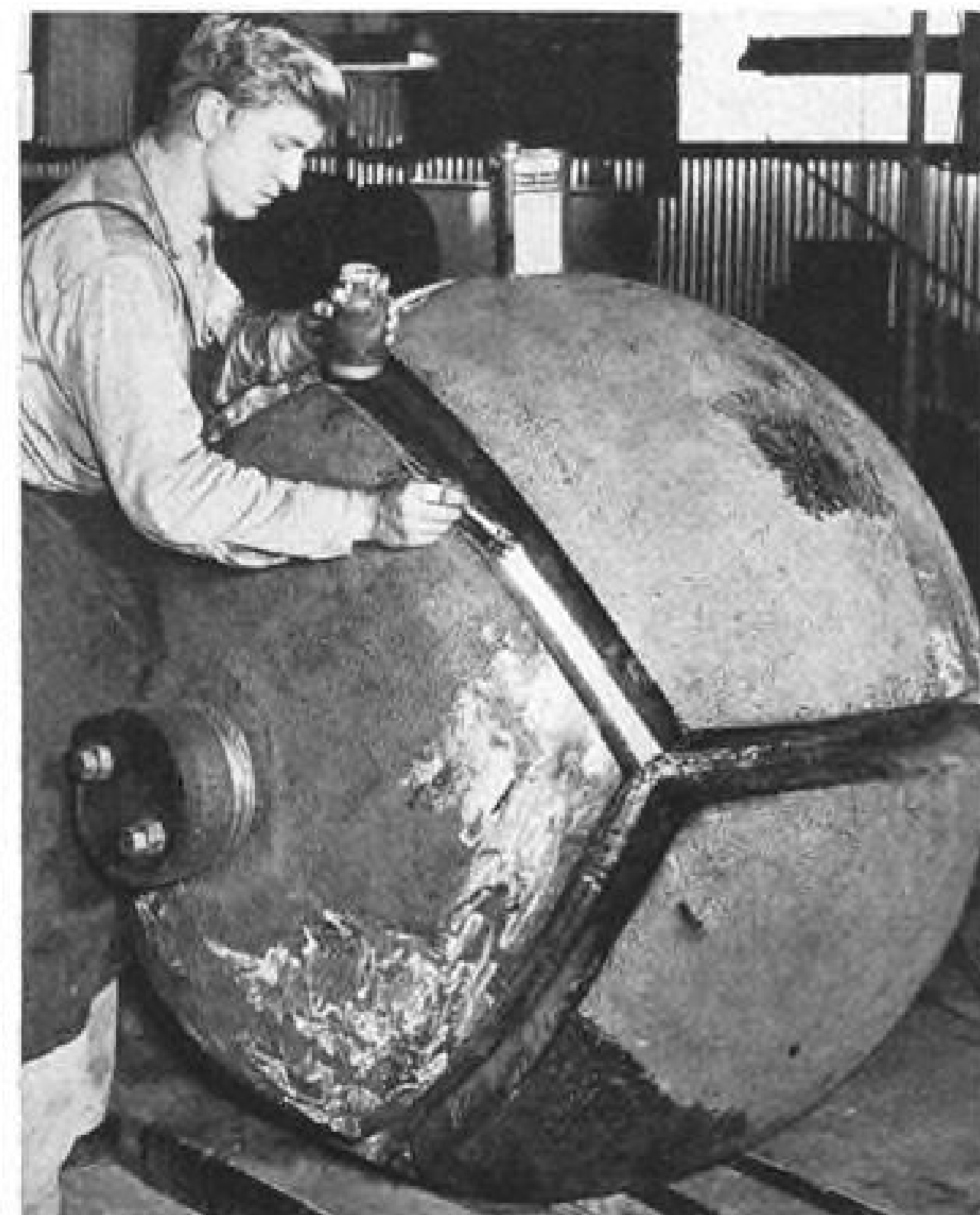
INSPECTING with Dy-Chek, a red surface-penetrant highlighted with developer.
