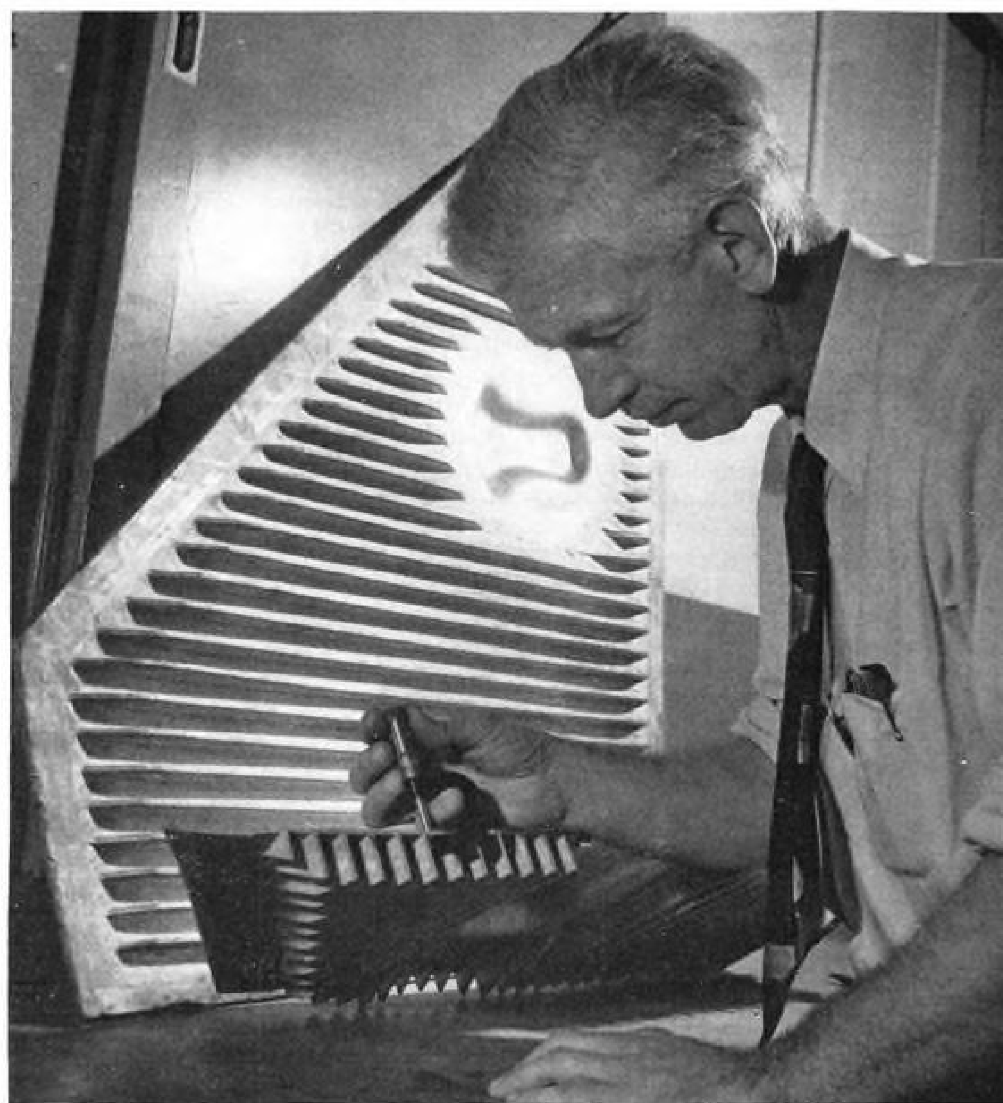
INTEGRALLY STIFFENED skin section, forged in one piece on Wyman-Gordon Co.'s 18,000-ton Mesta press, replaces part usually made of 25 individual pieces.
