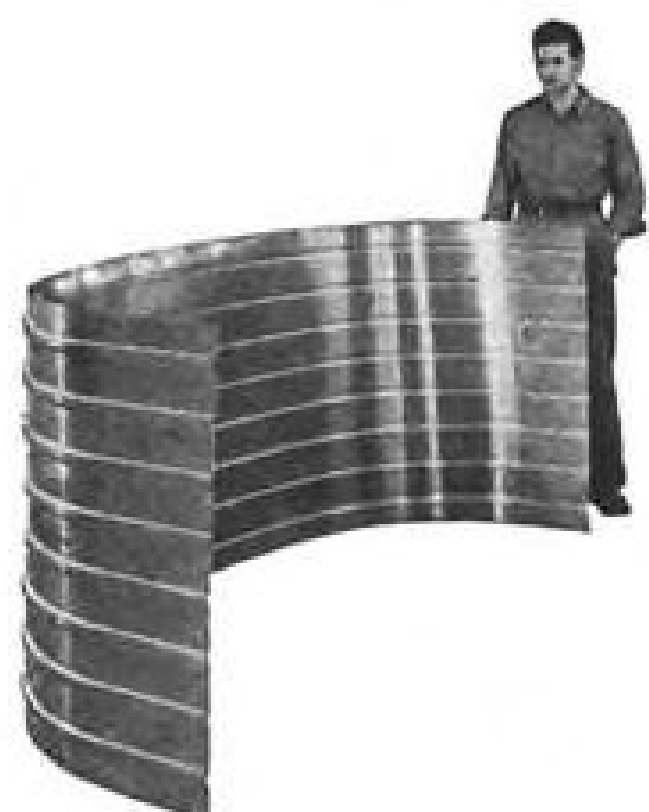
Large corrugated aluminum sheets accurately formed on the BATH machine.
