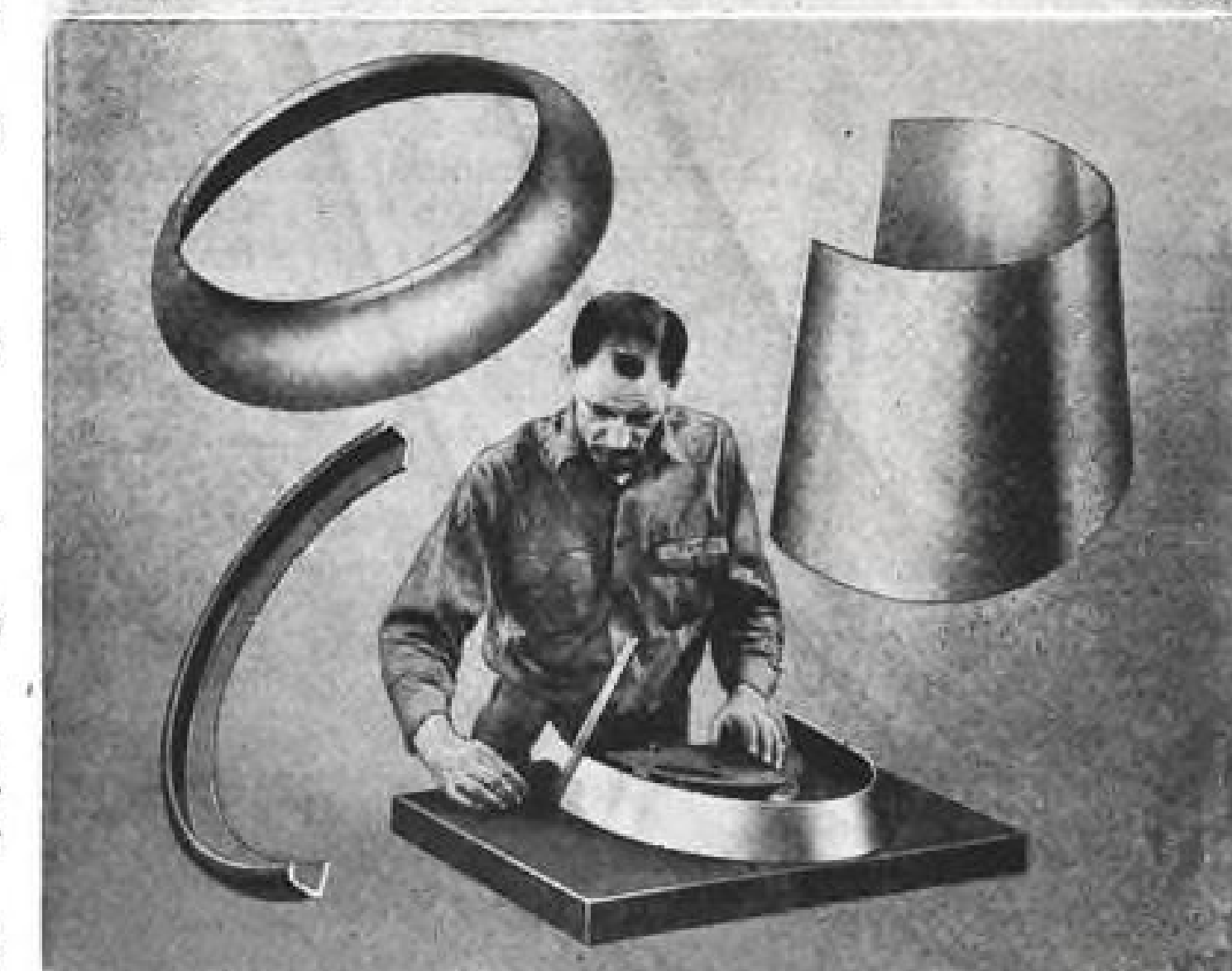
Above: Jet flange rings, shrouds, cases, flame tubes, stiffeners and casings are formed in either full circles or segments.
