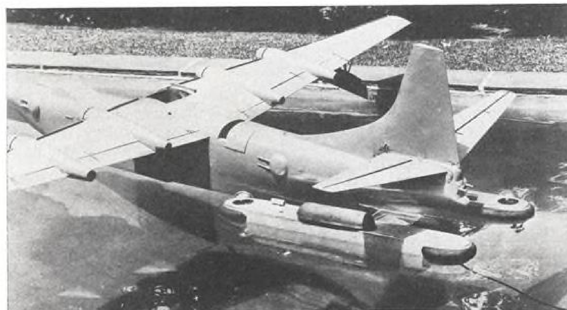
FLYING BOAT STERN. Pneumatic cushions rise to support plane underwing before . . .
