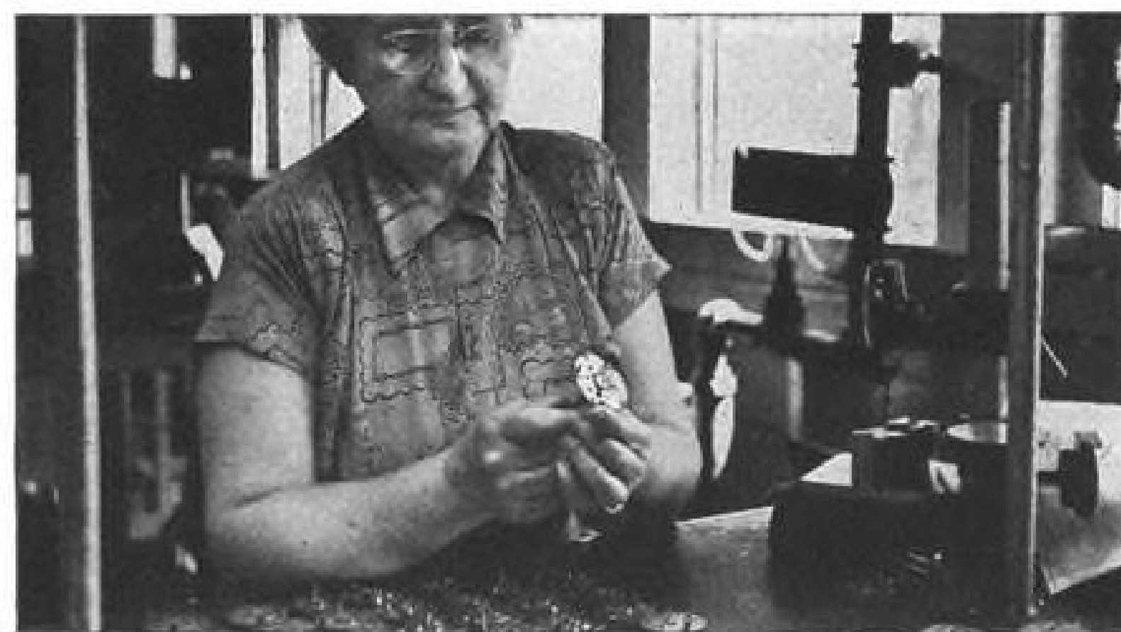
FINISHED PARTS are checked right on the assembly floor with plug gage standard pictured at left. Tolerances as close as 0.0001 in. are maintained.
