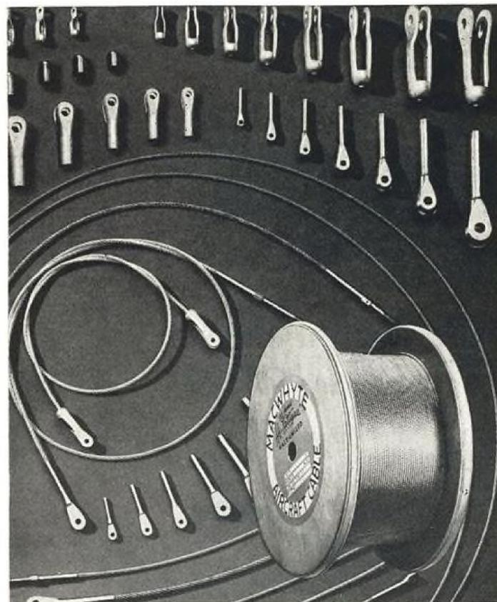
Macwhyte "Hi-Fatigue" Aircraft Cable is supplied in reel lots, specified lengths, and cable assemblies. Macwhyte "Safe-Lock" and "Socket-type" terminals are supplied loose or attached to cable.
