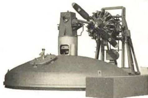
*Developed under Navy and Air Force contracts, the world's first supersonic spin pit is now in operation at the Aeroproducts Division of General Motors. This new technical advance permits study of new Aeroproducts spinning at supersonic rotational speeds.*
