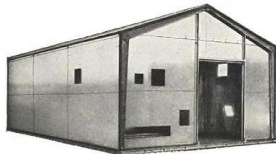
This portable shelter is made of honeycomb panels developed by the U. S. Plywood Corporation. All panels are attached with Simmons Roto-Lock Fasteners. Portable buildings are also being planned for alert hangars and maintenance hangars for fighter aircraft.
