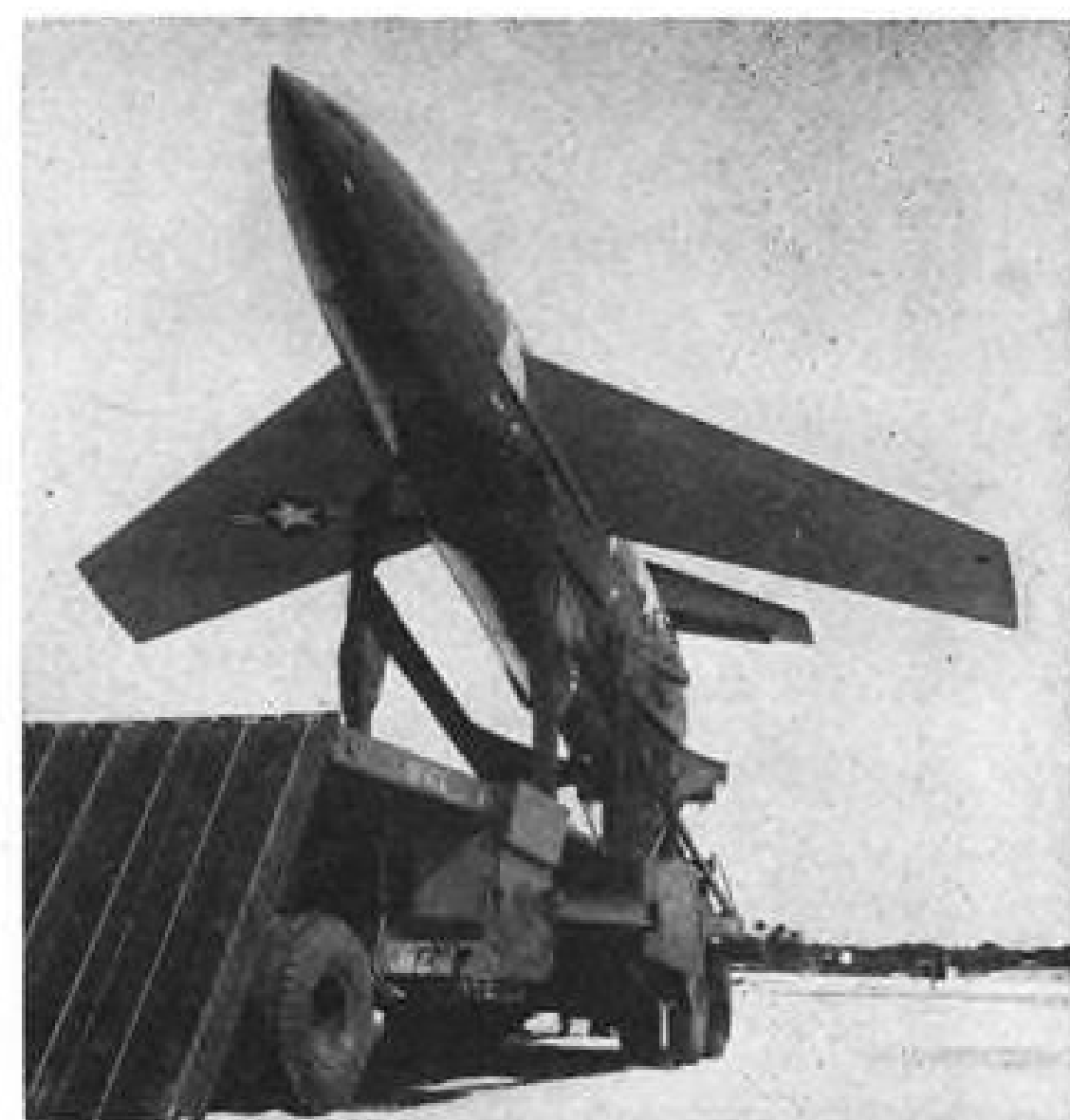
MARTIN MATADOR AF's B-61 missile, is poised on truck launching cradle. Weapon is about 30 ft. long, has thin swept wing. Basic power is supplied by Allison jet, but initial push is by RATO unit (arrow) as . . .
