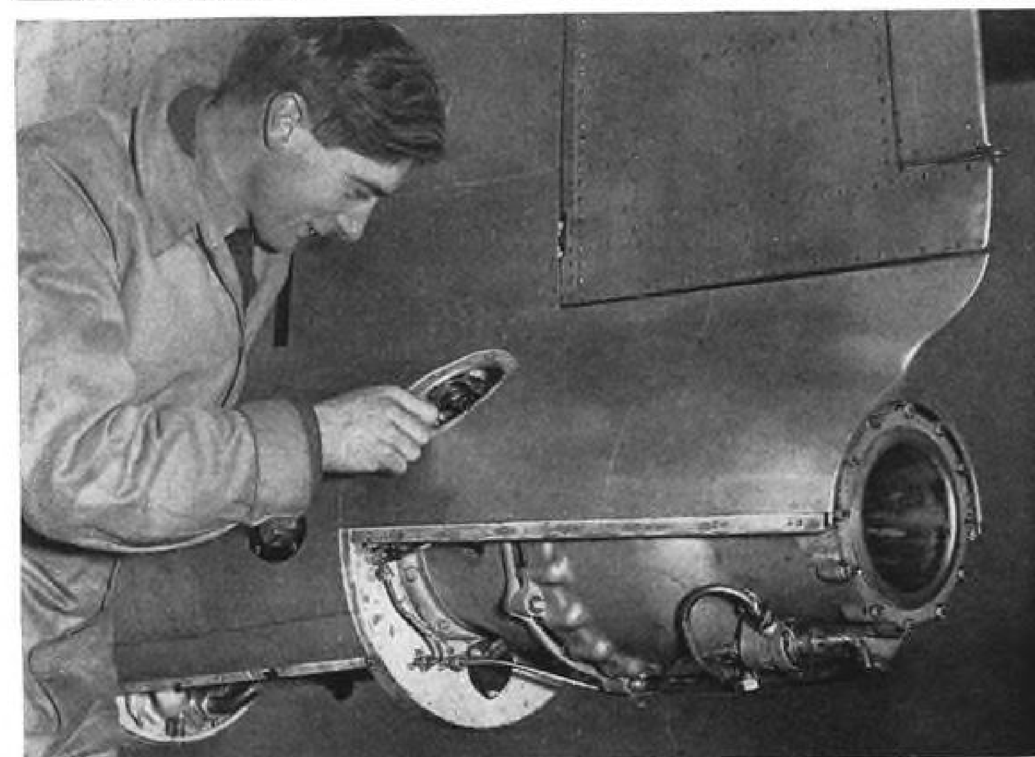
ROCKET MOTOR, fits into tail of jet fighter and provides auxiliary power in flight.
