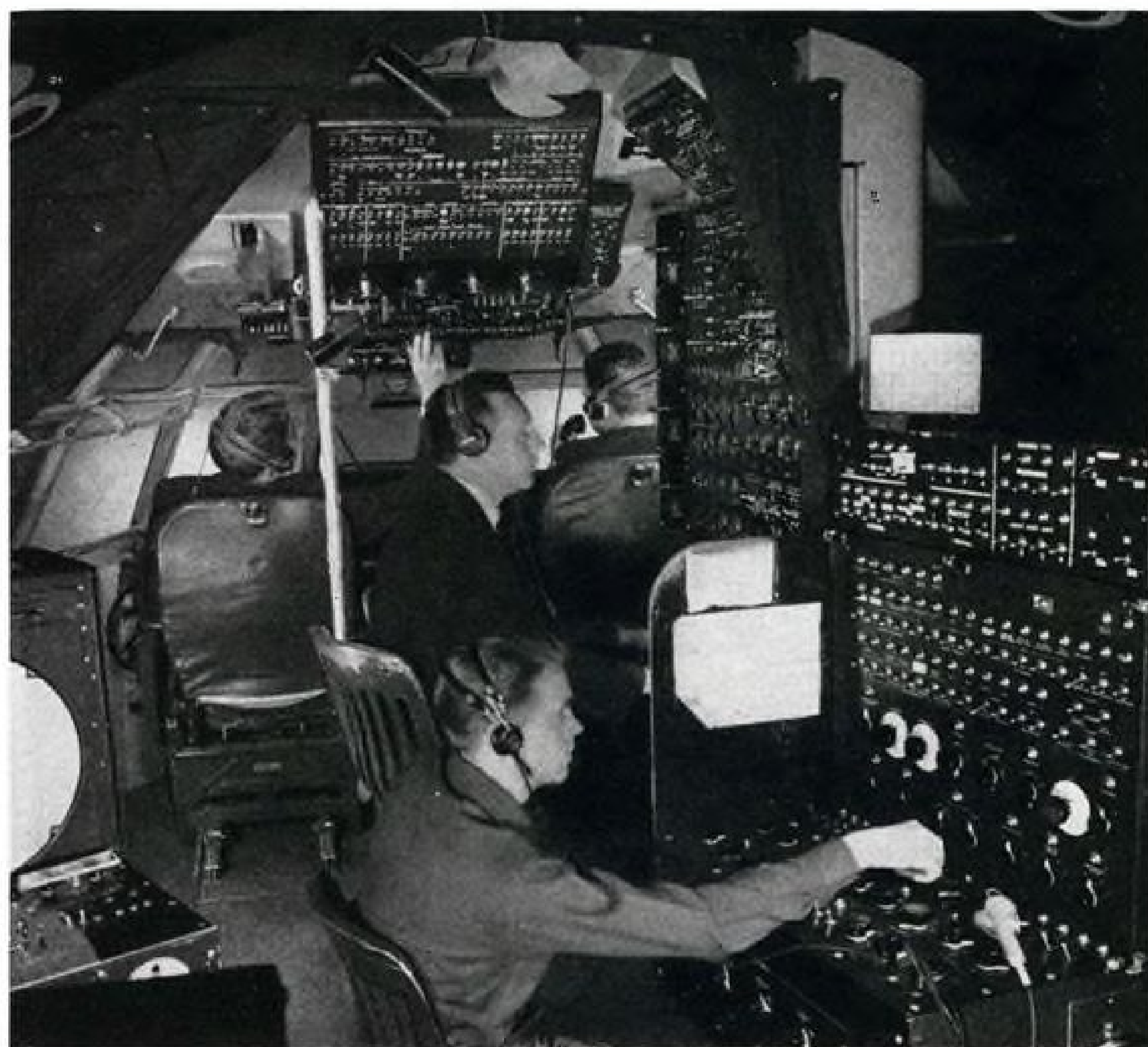
STRATOCRUISER simulator at PanAm with "flight condition" operator behind crew.
