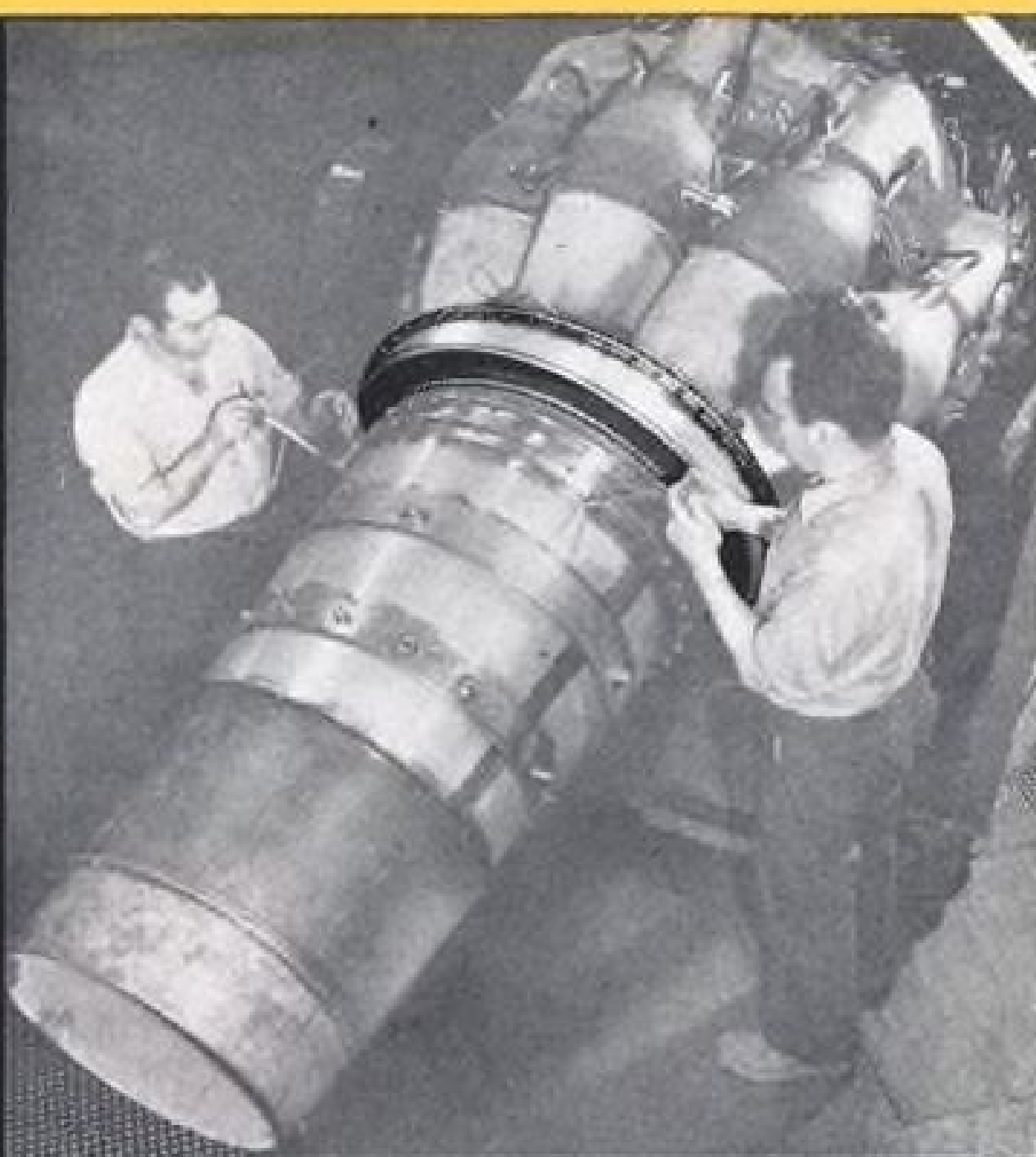
Hundreds of Air Manifold Cases for the Pratt & Whitney J-48 Turbo-Wasp are being turned out by Smith-Morris
