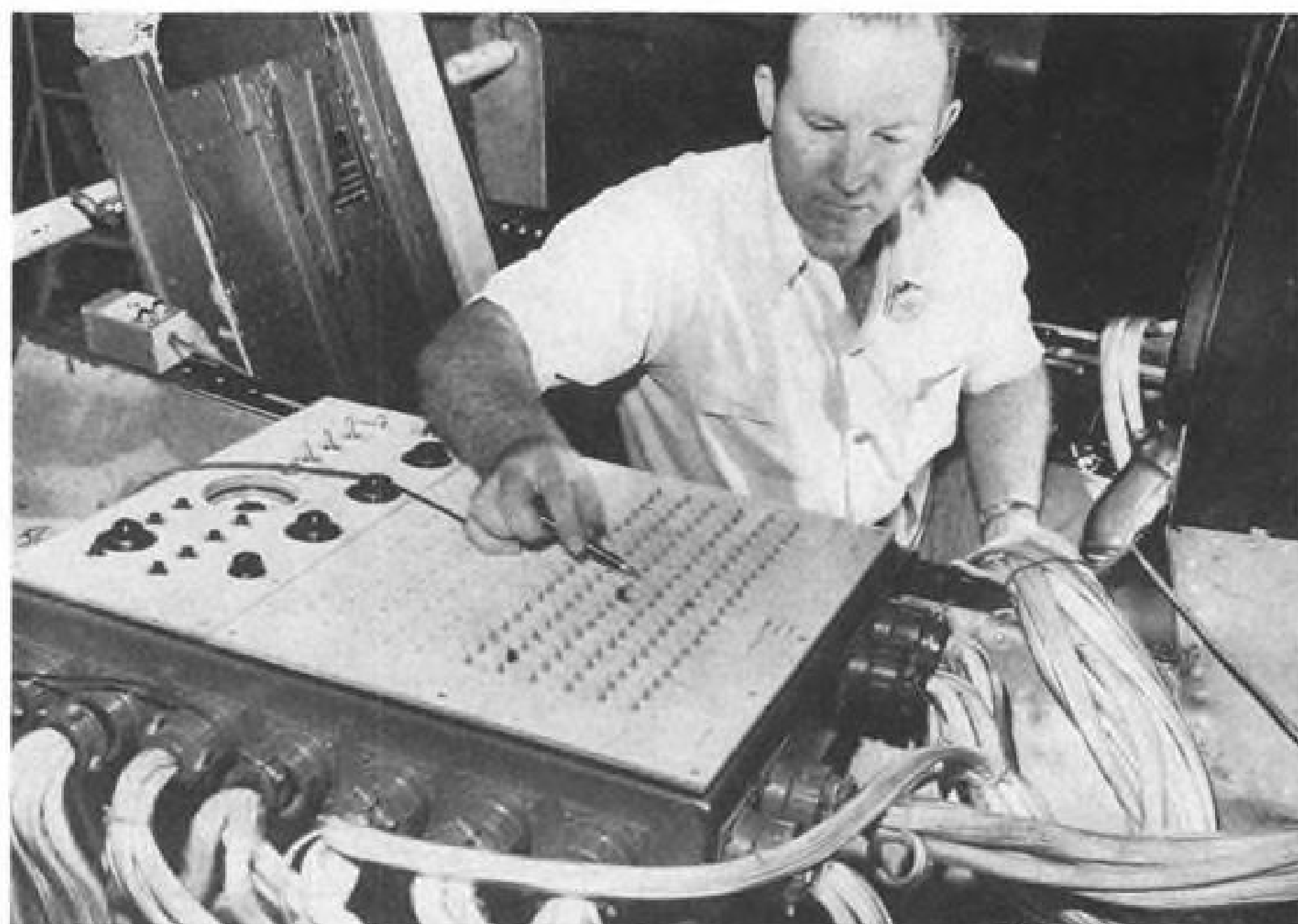
CONTINUITY CHECKER, with each post representing an electrical circuit, while . . .
