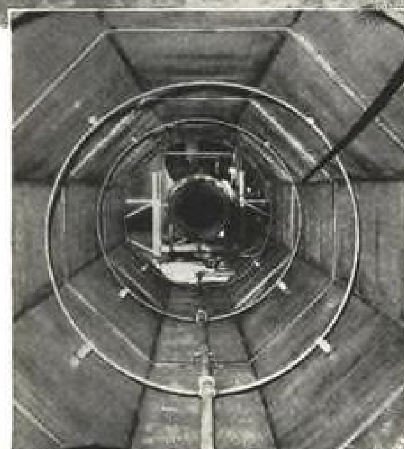
Interior of ISC Jet Aircraft Muffler.
