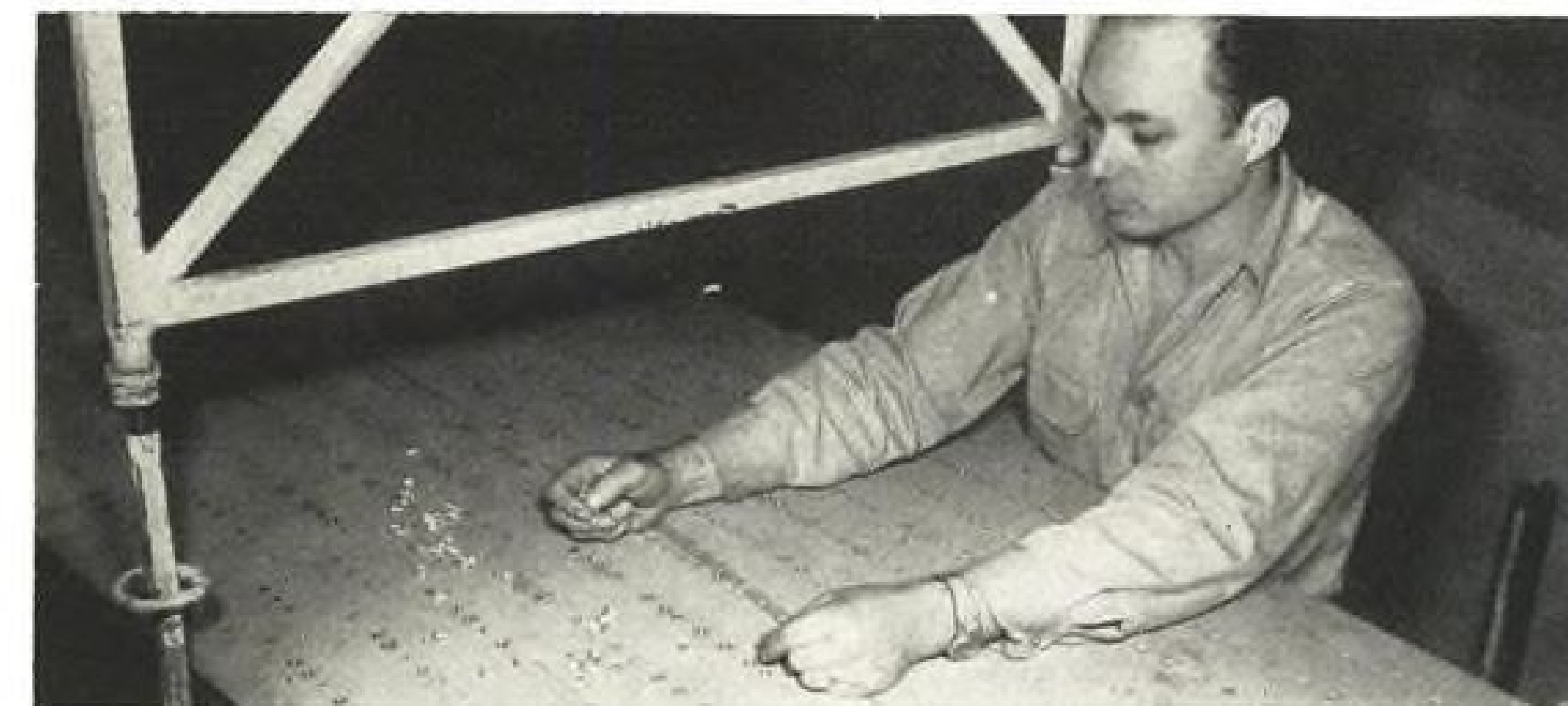
OLD METHOD of inserting the rivets by tedious hand process, and . . .
