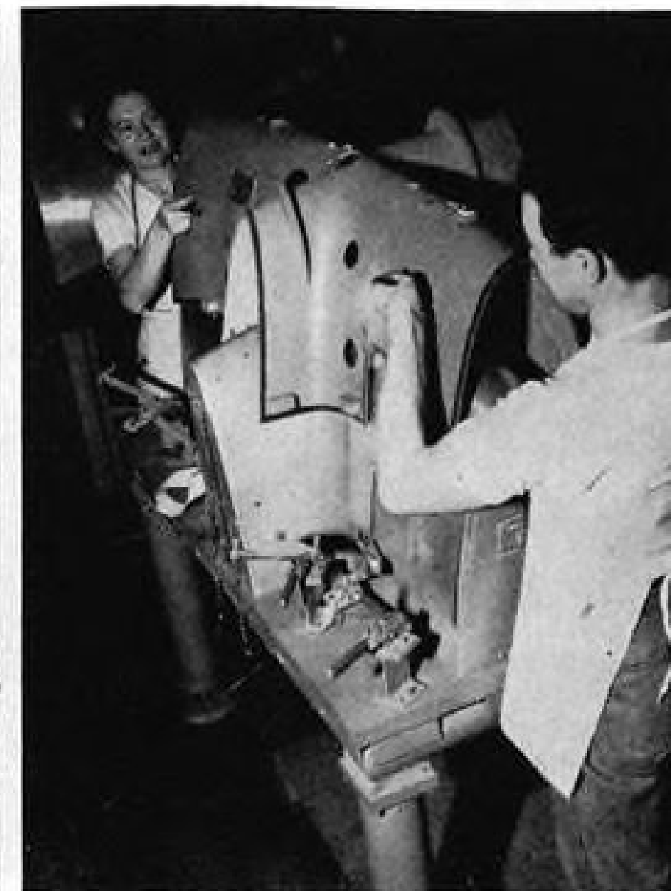
LOCKHEED technician installs gripper beads on plastic double-action die, while . . . WORKERS mount plastic drill guide.
