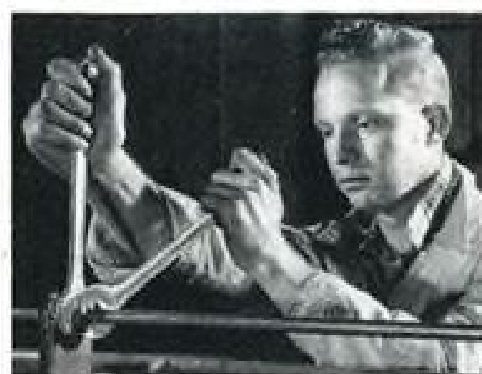
Tightening tail rotor shaft lock nuts, combination and open end wrench.
