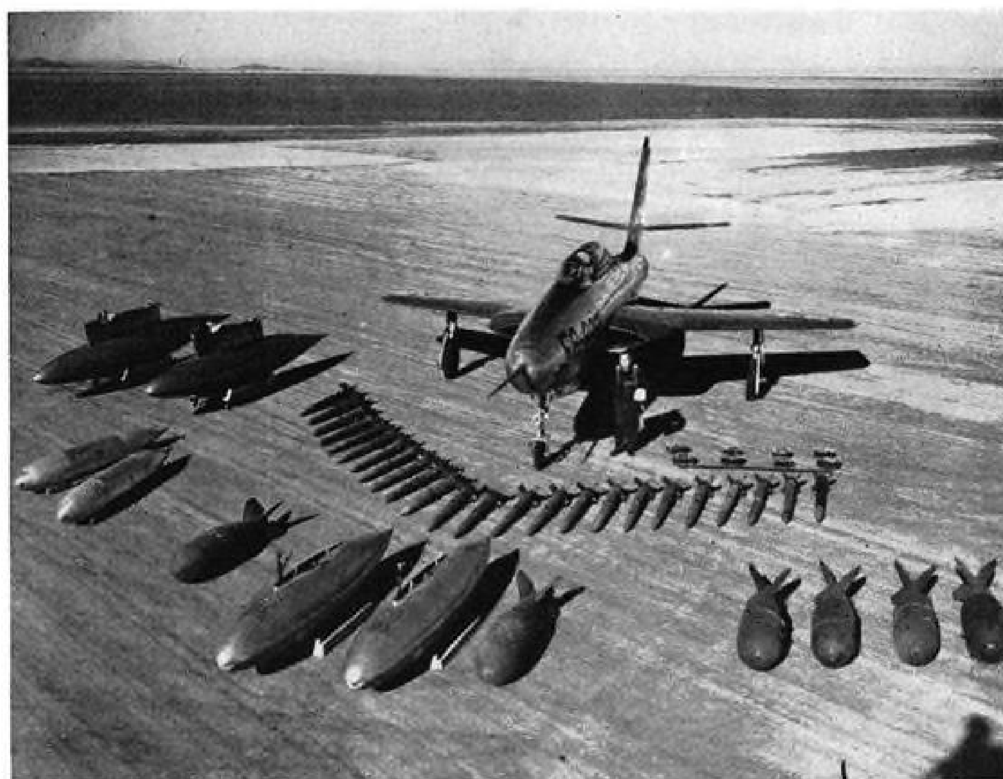
VERSATILITY is emphasized in new Republic F-84F. It can carry a wide variety of armament; some standard operational loads are illustrated above.
