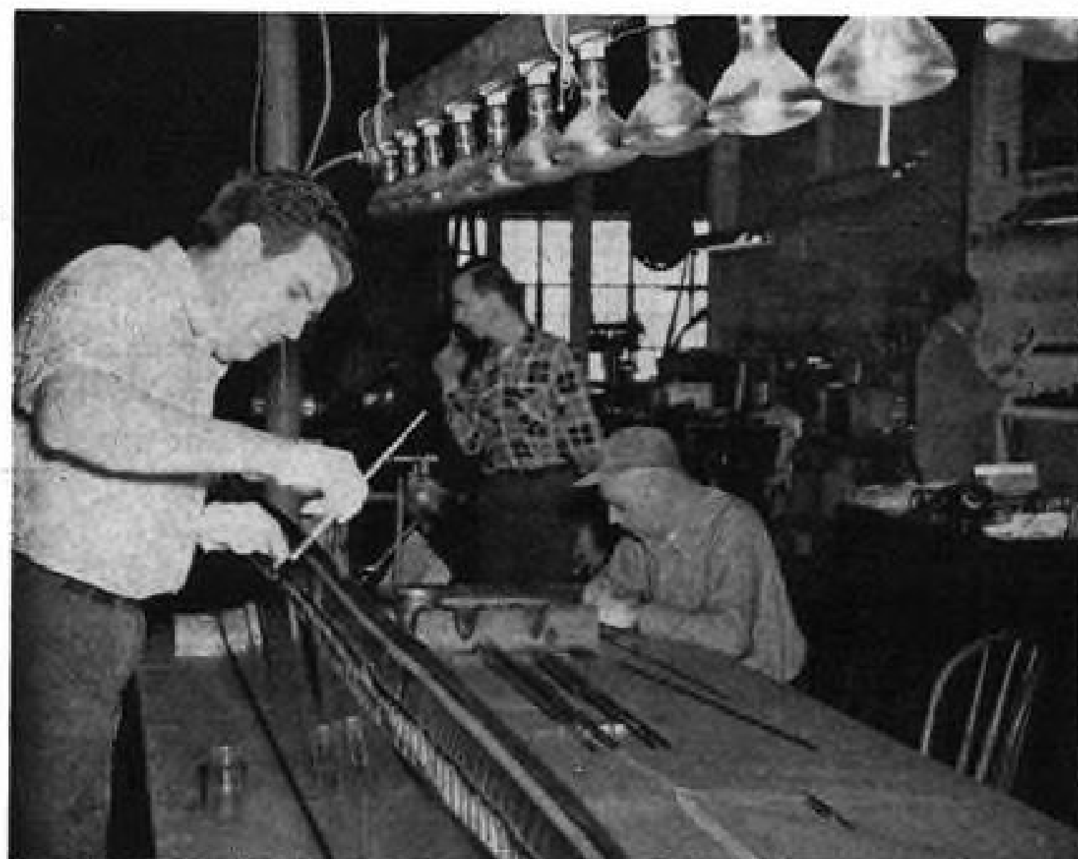
FINISHING coat of adhesive is applied to trailing edge after tacking.
