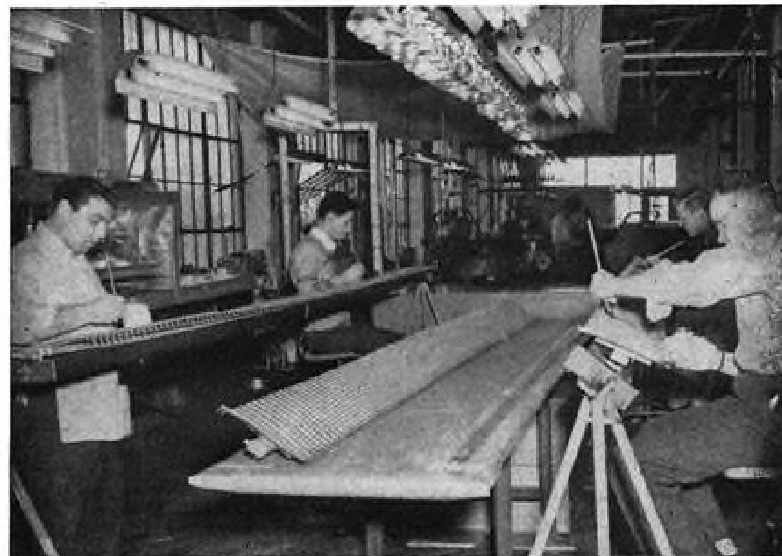
COATING of adhesive is applied by hand and paintbrush to the stamped stiffener.
