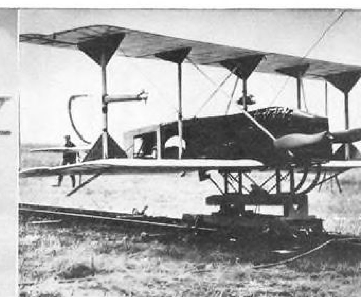
1916 Ancestor of the guided missile was the aerial torpedo developed during 1916-18 by Sperry working with the U.S. Navy. These automatically controlled "flying bombs" were tested over Great South Bay, Long Island.
