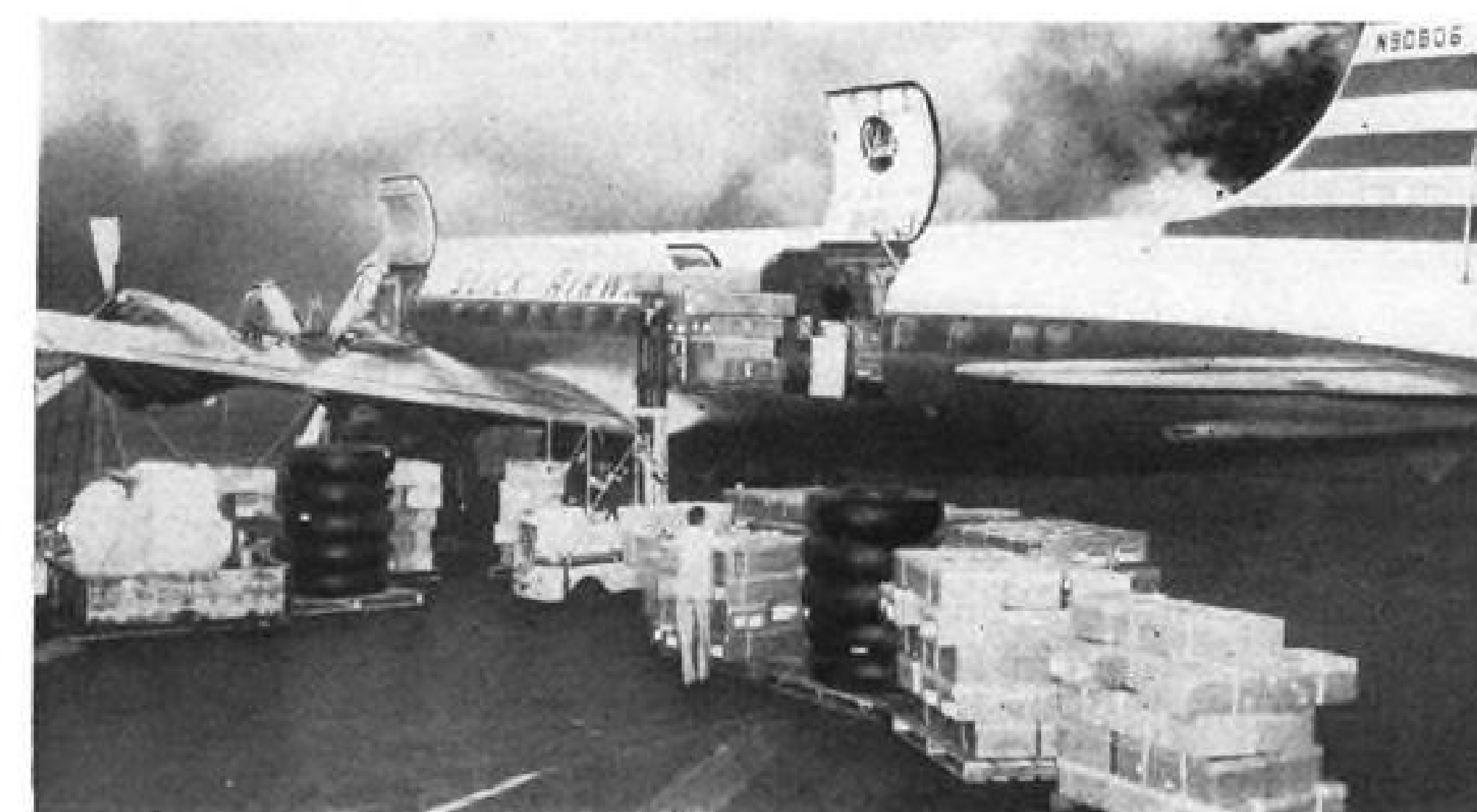
BIG LOADING DOORS make shipment of heavier and bulkier freight easier.
