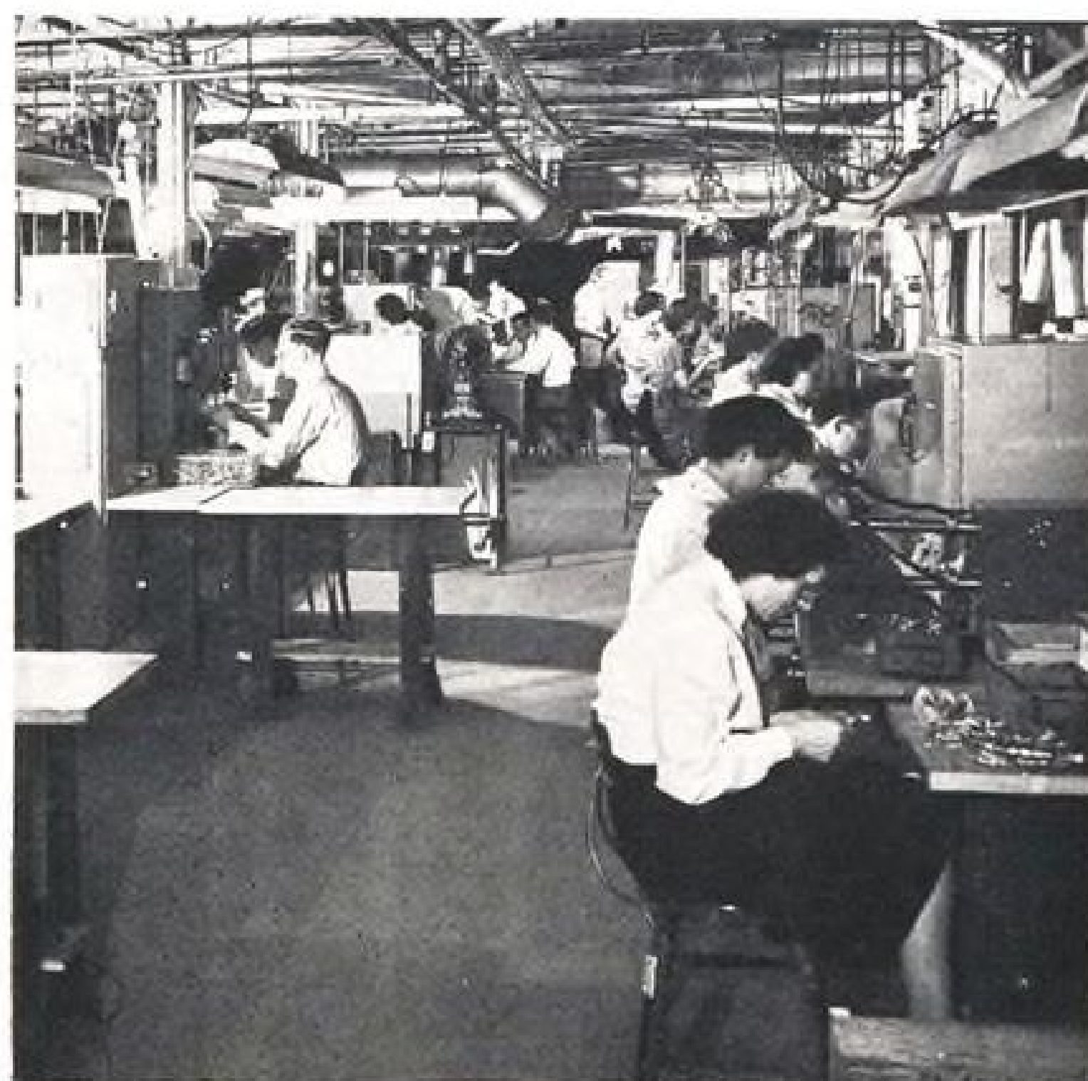
QUANTITY PRODUCTION of Fenwal Aircraft Heater Controls (as shown in this picture) is accomplished by well-trained assemblers who make up this assembly line. Their skill is backed up by rigid quality control methods which include X-ray inspection. Adequate and efficient production facilities keep all Fenwal THERMOSWITCH units moving in increasing quantities.
