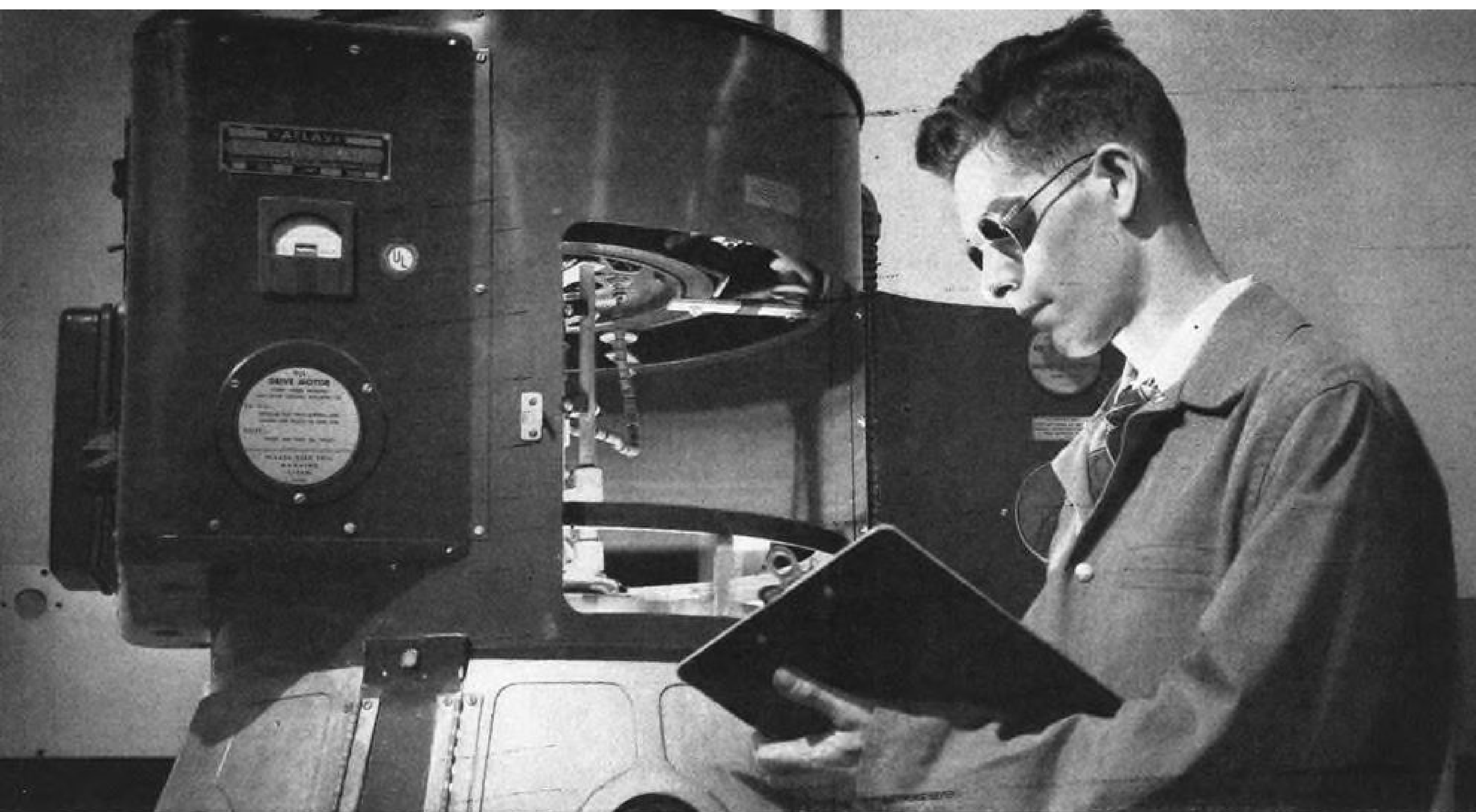
INSTRUMENTS ARE EXPOSED TO ULTRA-VIOLET RAYS TO DETERMINE THE EFFECT OF SUNLIGHT ON LEGIBILITY OF DIALS
