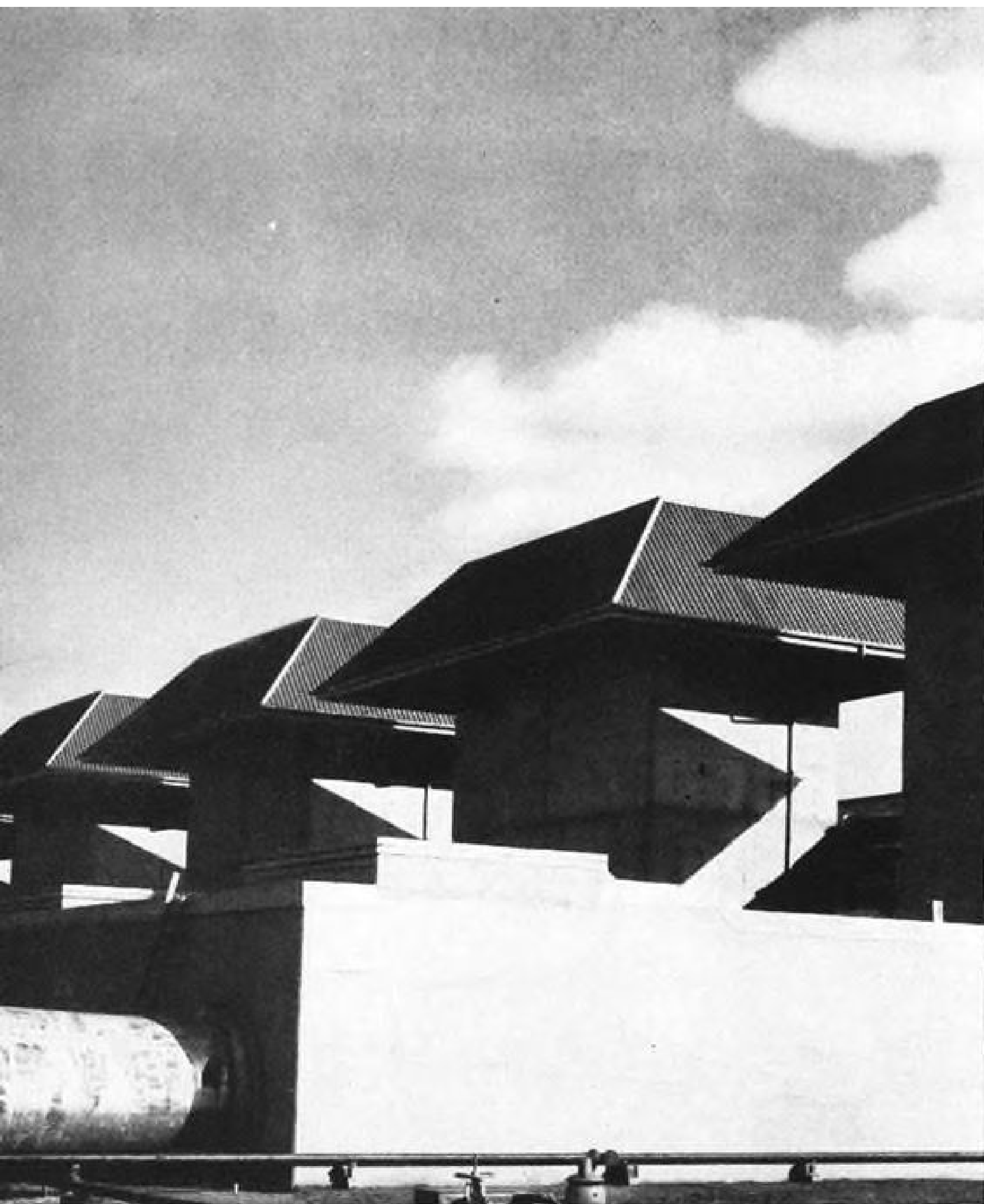
LOCKLAND PRODUCTION ENGINES are tested in 33 fortress-like cells. Exhaust stacks withstand 1000+°F temperatures and have excellent sound absorption qualities.
