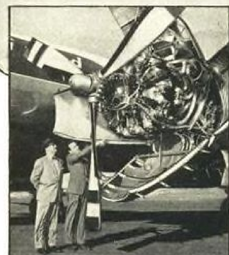
Pratt-Whitney R-2800 CB-16 Engines pack the power—and these new lightweight, low-cost Lord Mountings increase the payload approximately 10 lb. per engine... protect the air-frame from vibration... give passengers a smoother ride.
