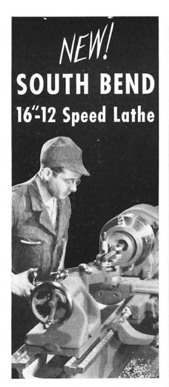
This new South Bend Twelve-Speed Lathe will save time in the production shop, toolroom, maintenance, or wherever an extra wide range of spindle speeds is needed. Equipped with pushbutton control which provides instantaneous changes between high and low speeds, multiple operations requiring frequent speed changes such as drilling and tapping, boring and reaming, or turning and facing can be performed with utmost efficiency. Write for catalog.
