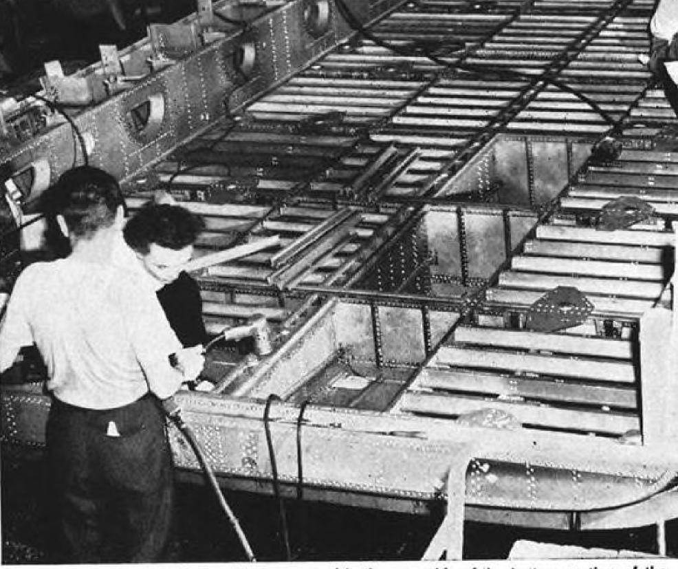
Du Pont Aircraft Explosive Rivets are used in the assembly of the bottom section of the fuselage of a C-119 Aircraft made by Fairchild Aircraft Division of Hagerstown, Maryland.
