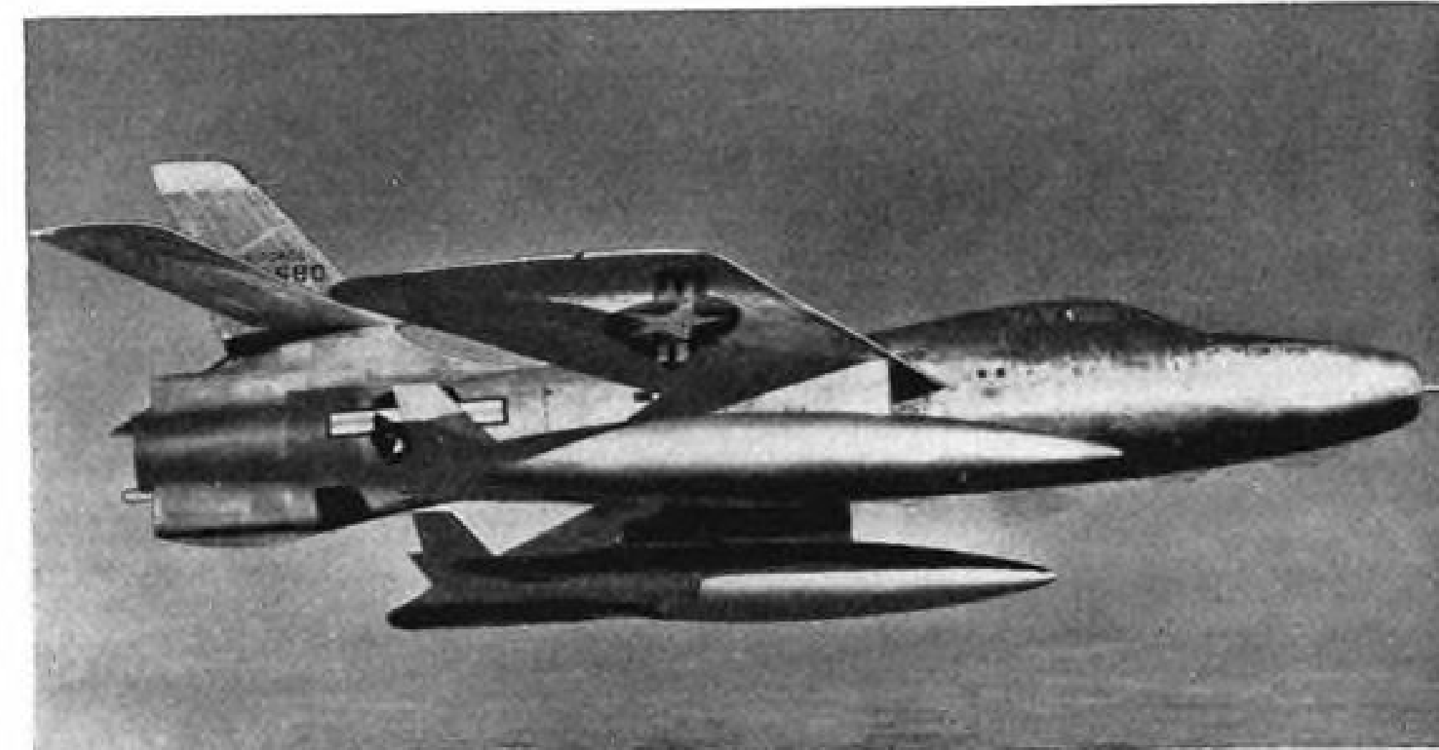
REPUBLIC XF-91 has four Reaction Motors rockets above and below J47 tailpipe.
