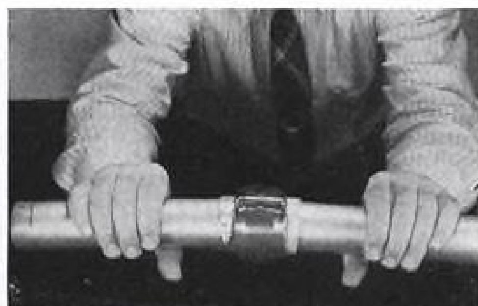
FLEX JOINT for rigid tubing will find application in the B-47, where it will accommodate fuel lines to the Stratojet's 20-ft. wing deflections.
