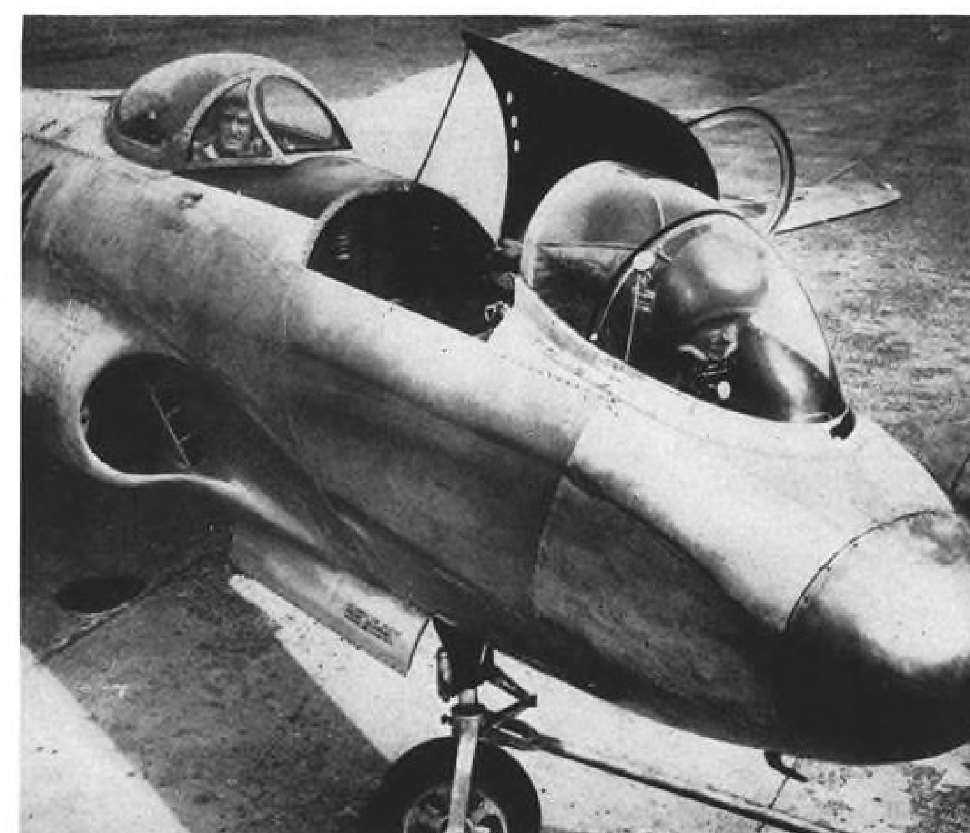
MODIFIED F-80E had prone position in its nose. Pilots found it comfortable.
