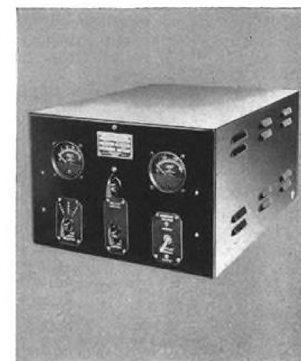
J&H Model GC23-20 Control Panel—closely regulates generator output.
