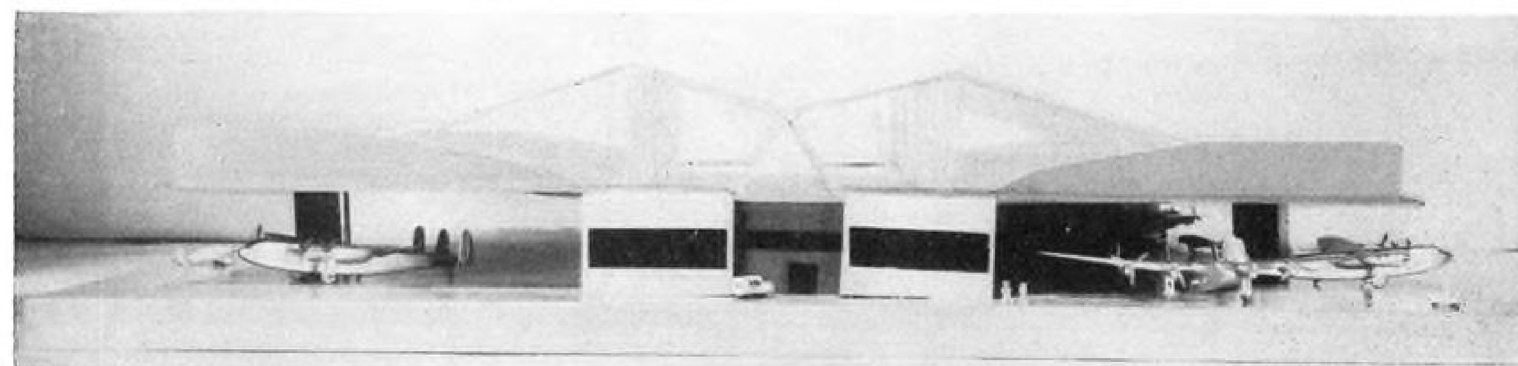
UNOBSTRUCTED FLOOR SPACE which can be used for large-scale production overhauls. Double unit is pictured.
