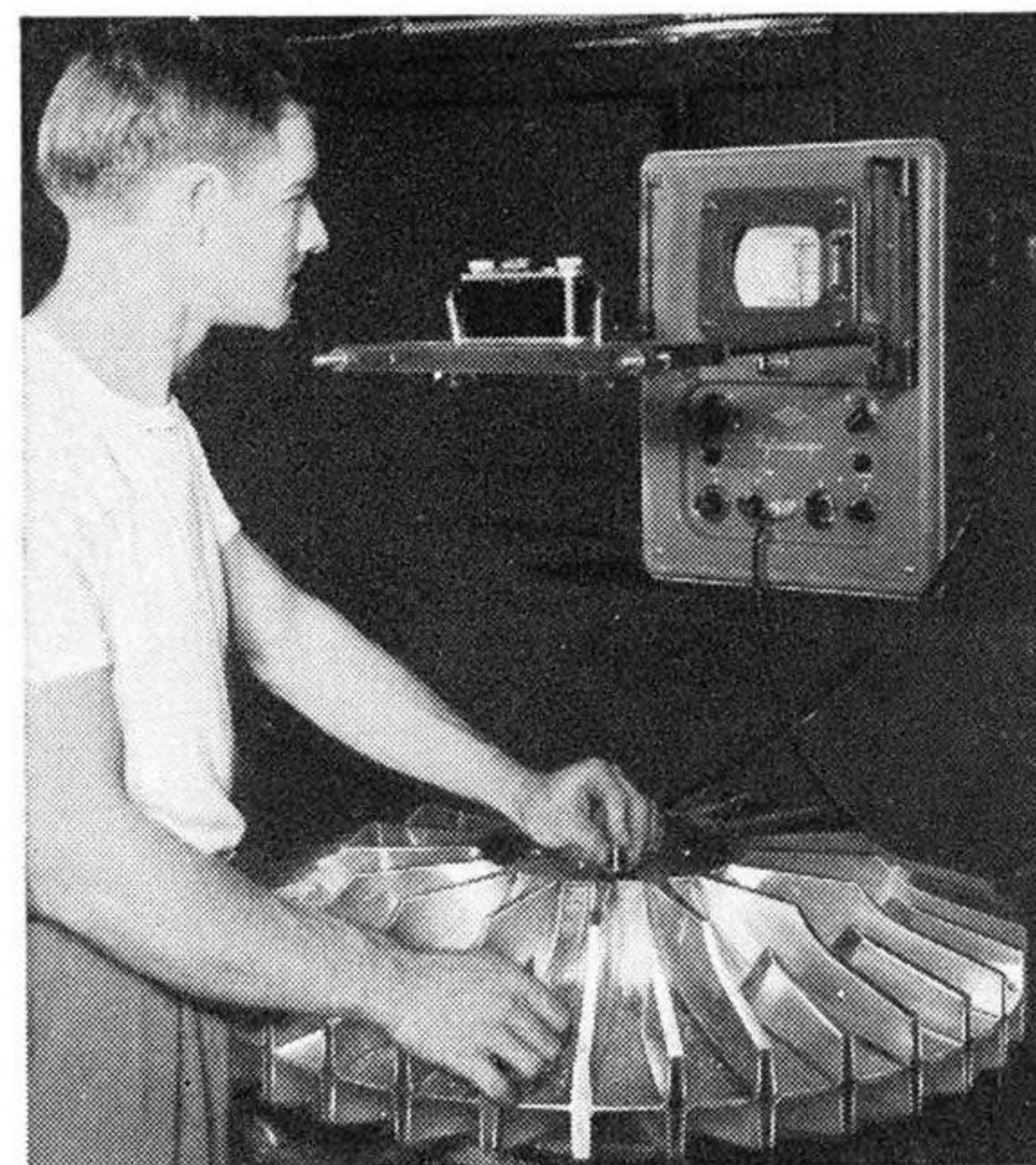
Several engine pieces, like this J33 compressor, receive 100% Ultrasonic inspection
