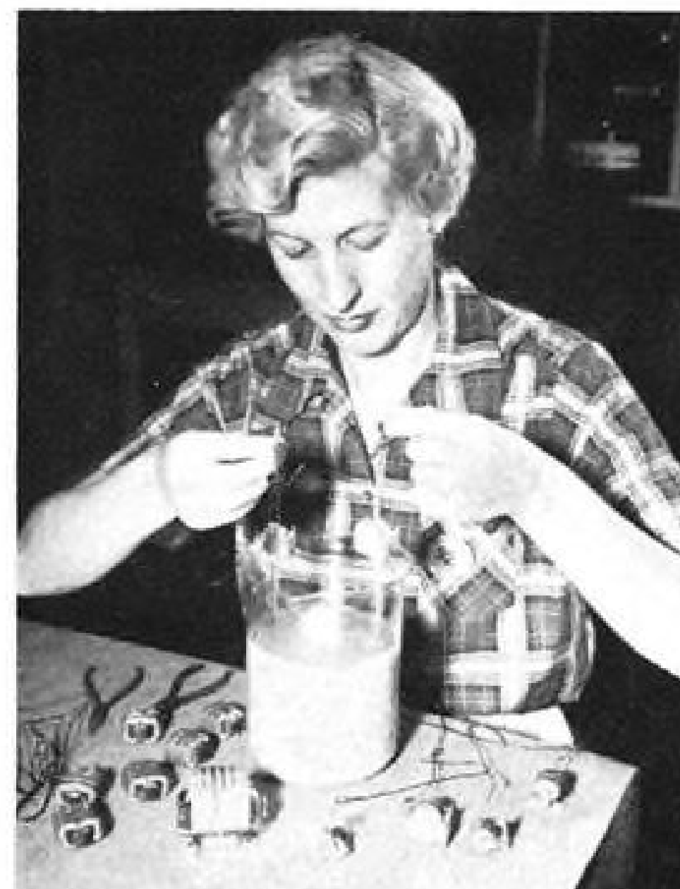
POTTING in resin to hermetically seal it.
