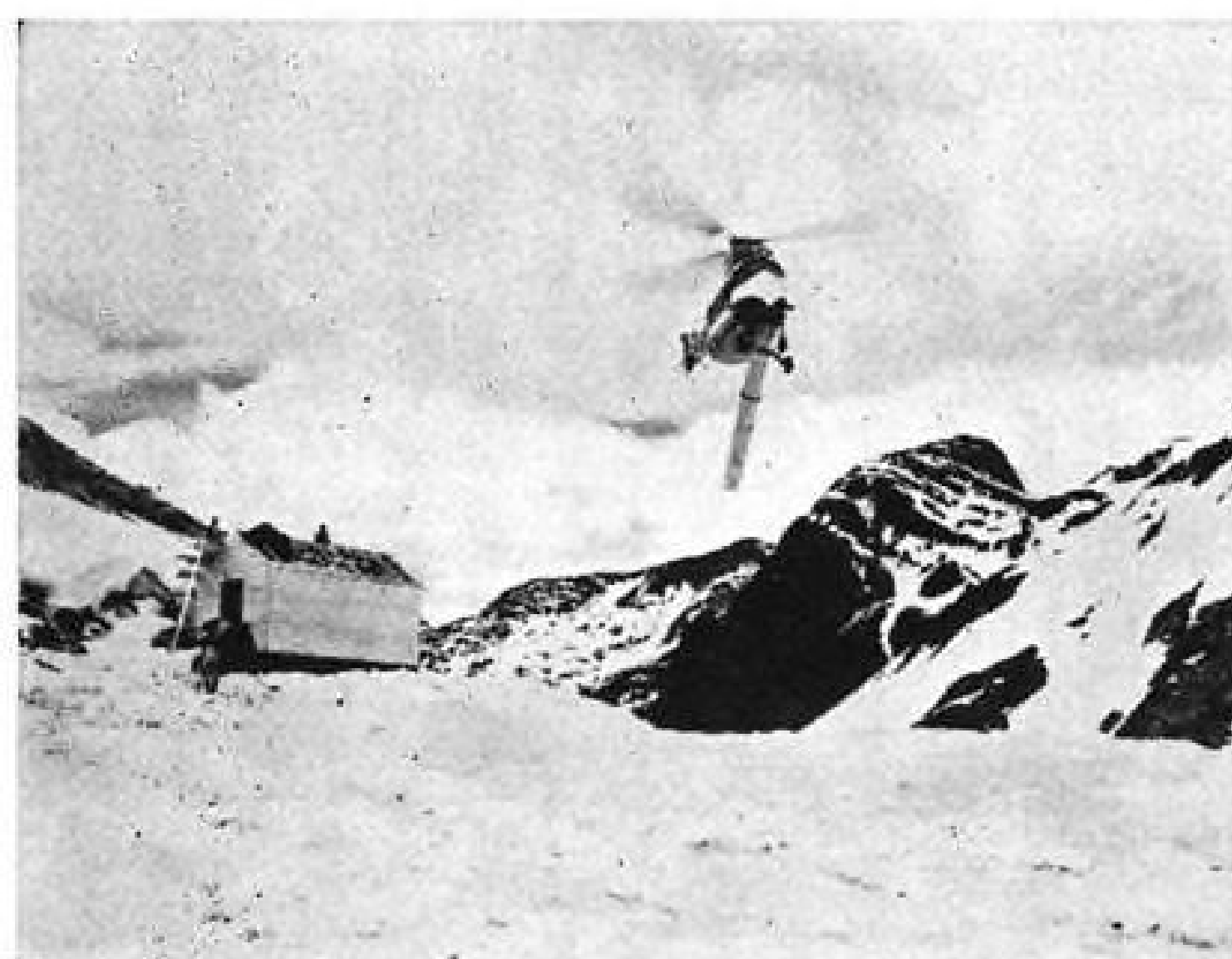
HIGH HAUL —In rugged British Columbia, a 50-mile power line is being built to serve an Aluminum Company of Canada plant at Kitimat. Work on this project has been enormously speeded by S-55s, flown by Okanagan Helicopters, Ltd., which can airlift almost everything needed to virtually inaccessible construction sites.
