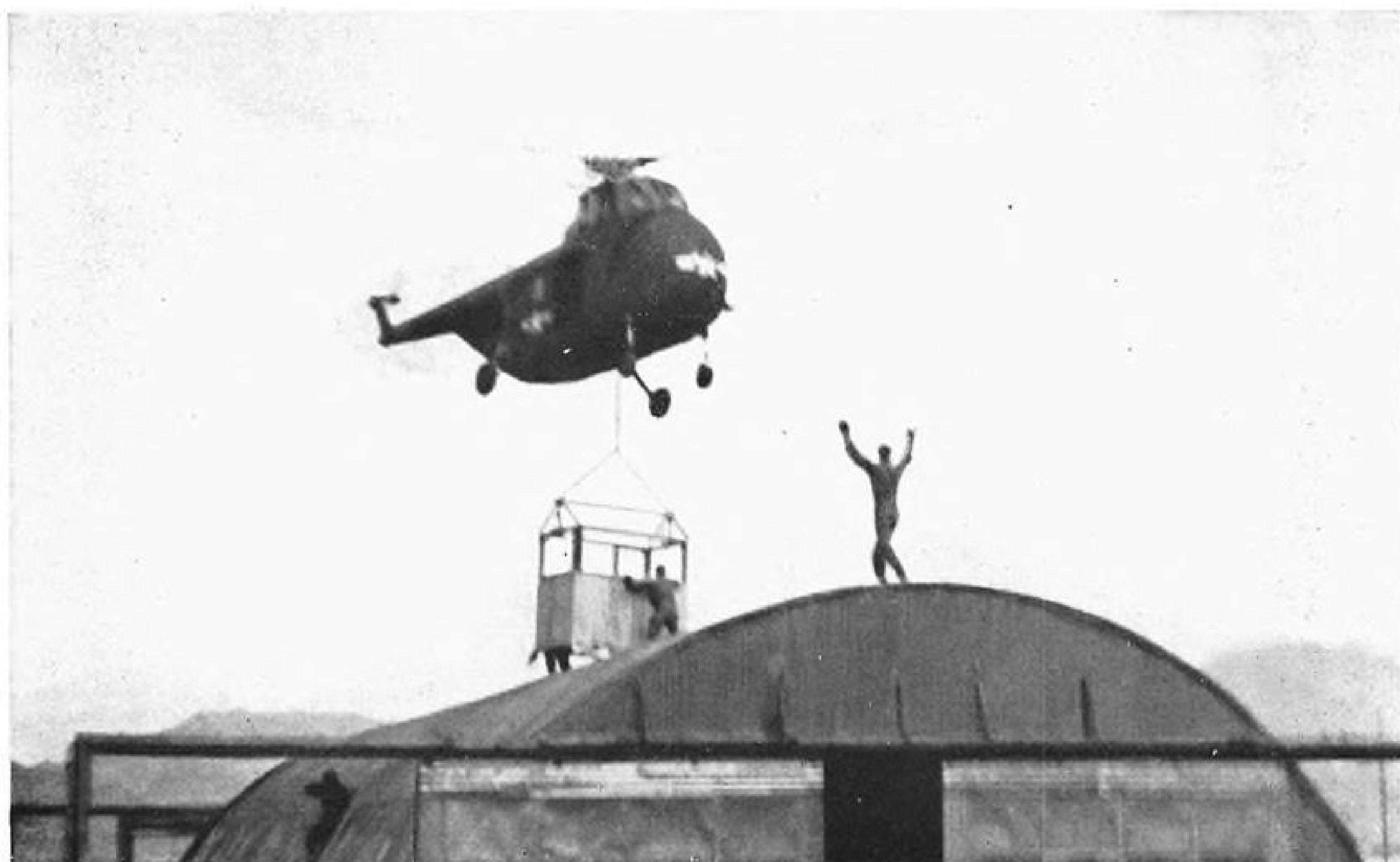
FIELD EXPEDIENT —It required only a few minutes for this big Army H-19 Sikorsky helicopter to lift and place a prefabricated control tower into position atop an airfield-
