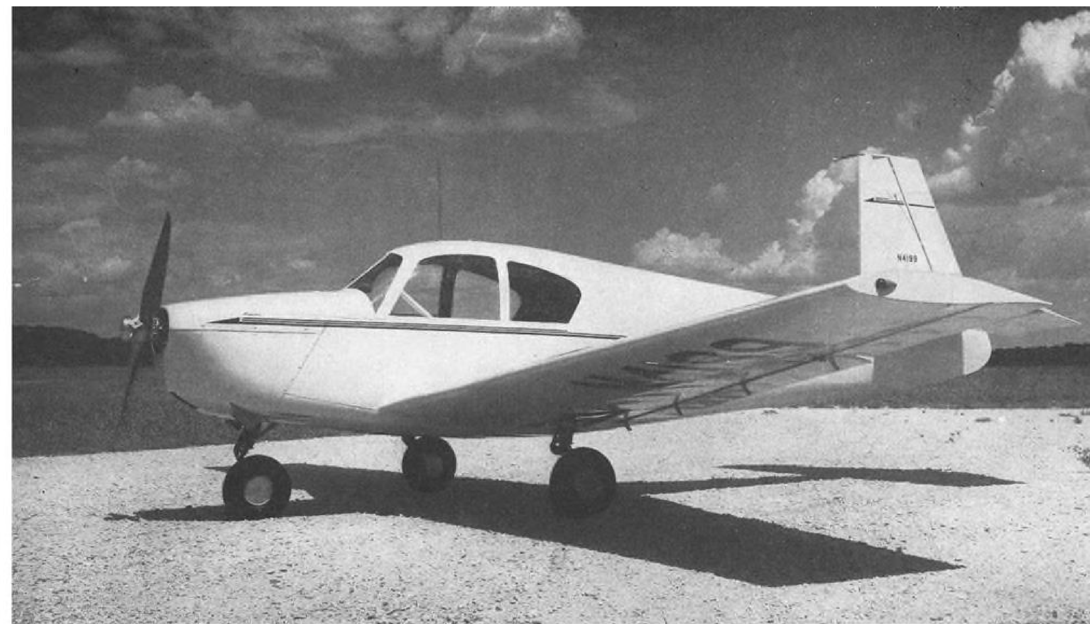
MOONEY FOUR-PLACER FLIES —First photo of new Mooney Model 20 Scotsman four-seat personal plane which made its first flight Aug. 10 at Kerrville, Tex. The plane is powered by a 145-hp. Continental and cruises at more than 160 mph.
