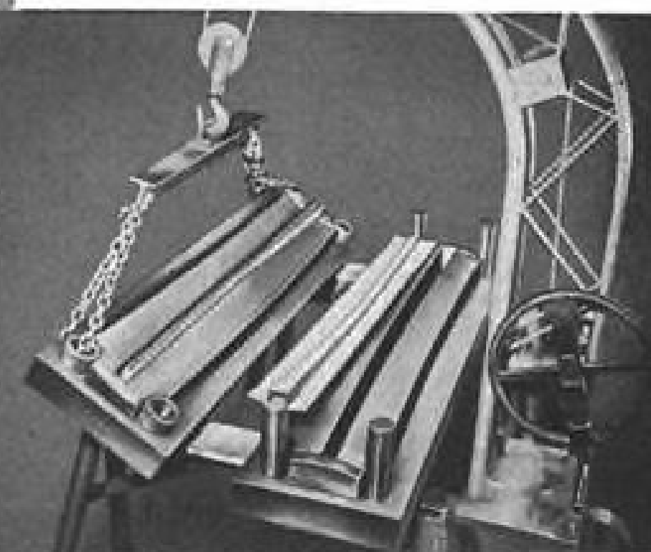
TWIX made Die to make a Hat-Sectioned Longeron in one operation. Longeron Dimensions: 72" long x 7" wide having Double Contour.
