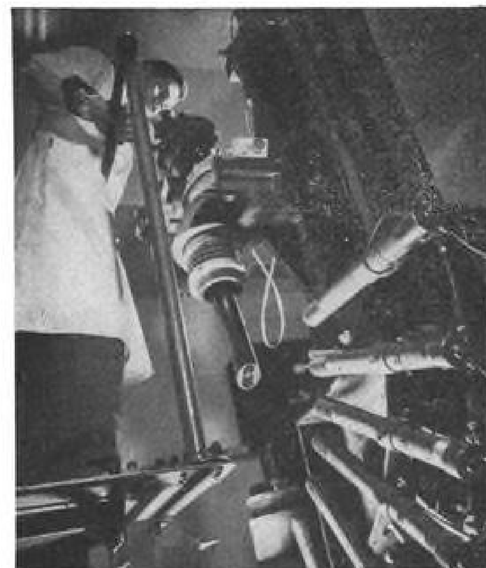
INSTRUMENT OVERHAUL is accomplished in air conditioned shop; at right, driftmeter is checked by technician.
