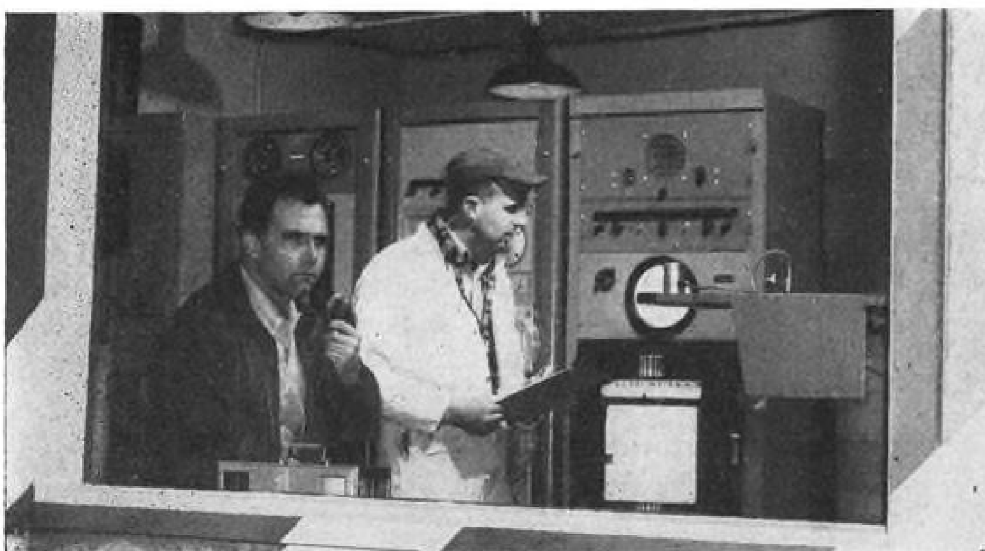
GROUND STATION remotely records weather readings and synchronizes them on tape recording with flight crew's observations on actual visibility conditions.
