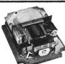
USAF Type T-1 High Interrupting Capacity Contactor
