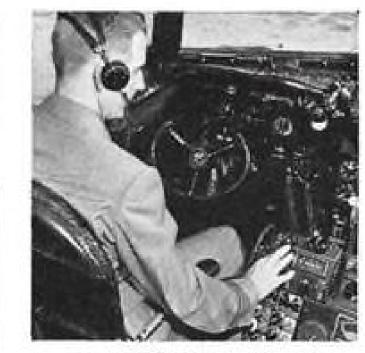
1946 United Air Lines installed Sperry A-12 Gyropilot on four-engine fleet to insure precise automatic instrument approaches to airport runway.
