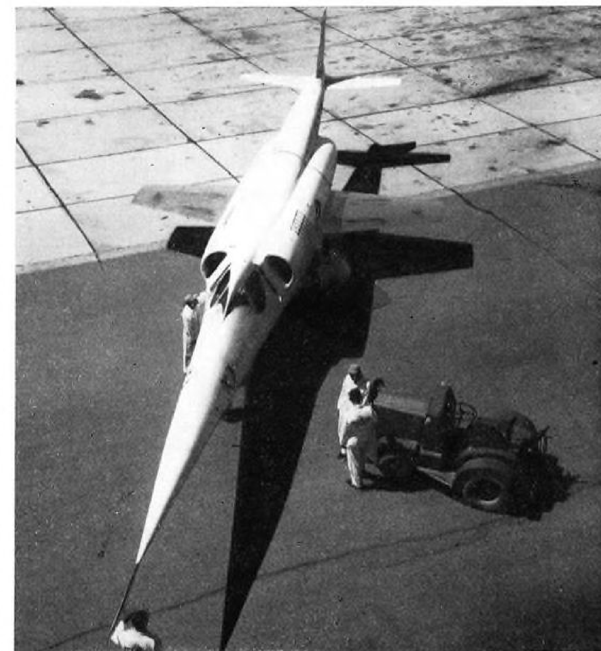
STUBBY WINGS, spanning only 22 ft. 8 in. are highlighted in this view of X-3.
