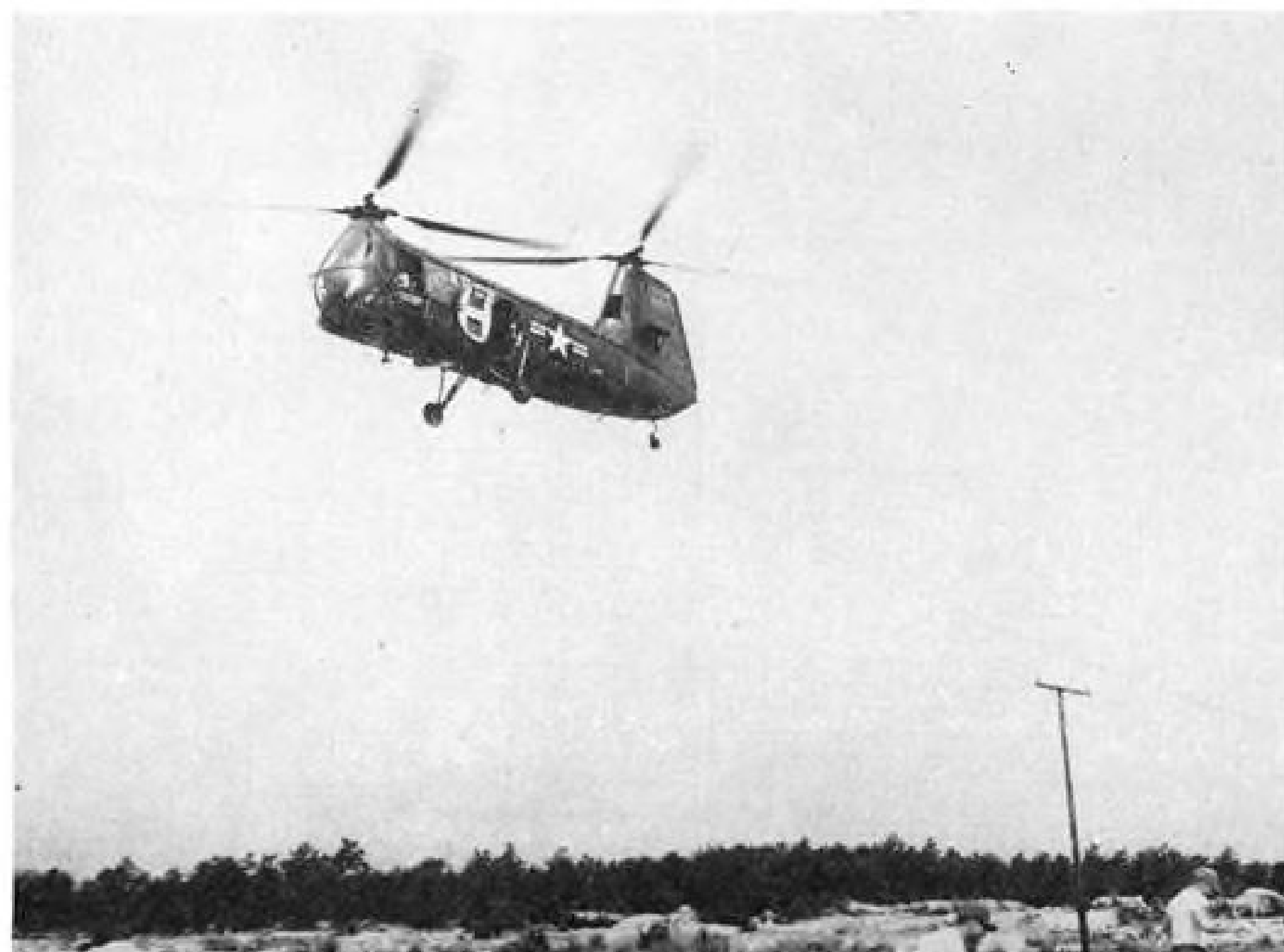
4 Flying sideways, a routine helicopter maneuver, the Army Mule accurately lays the phone cable directly onto the crossarms of the erected telephone poles.
