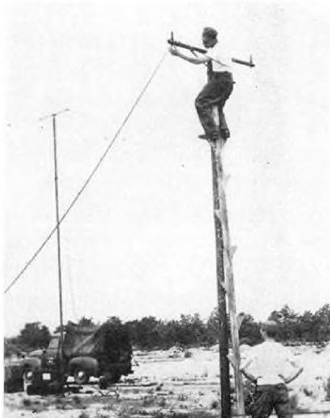
5 All the Signal Corps linesman has to do now is secure the cable to the pole's crossarm.
