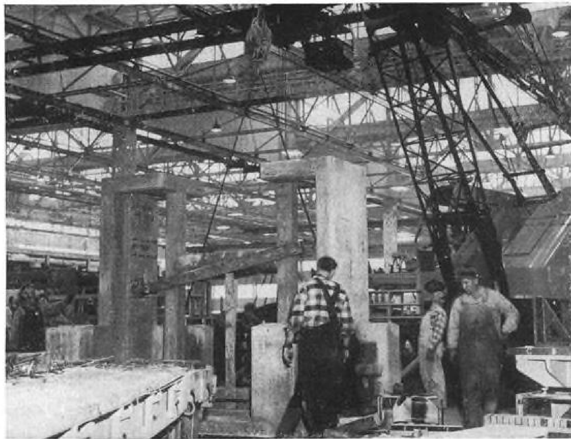
SOLID SUPPORT will be given steel jig by concrete base, shown going into place.
