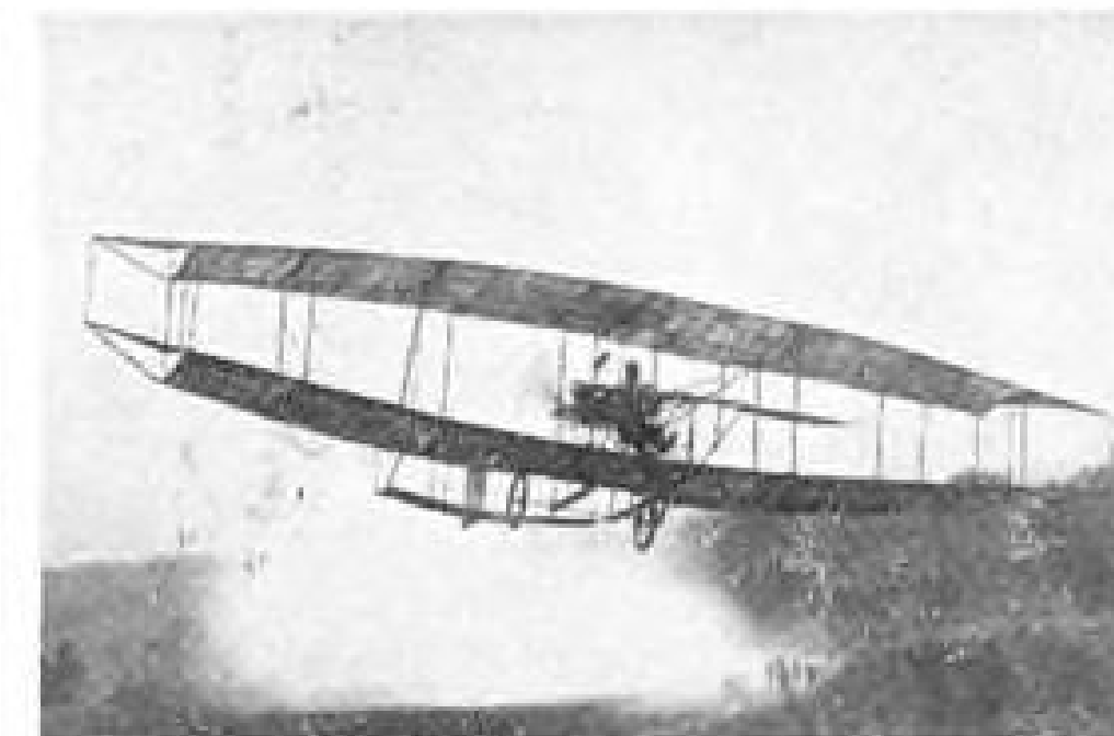
Glenn Curtiss first exploited lateral control effected by ailerons in 1908. In his pusher plane, the June Bug, he got off the ground at 150 feet!
