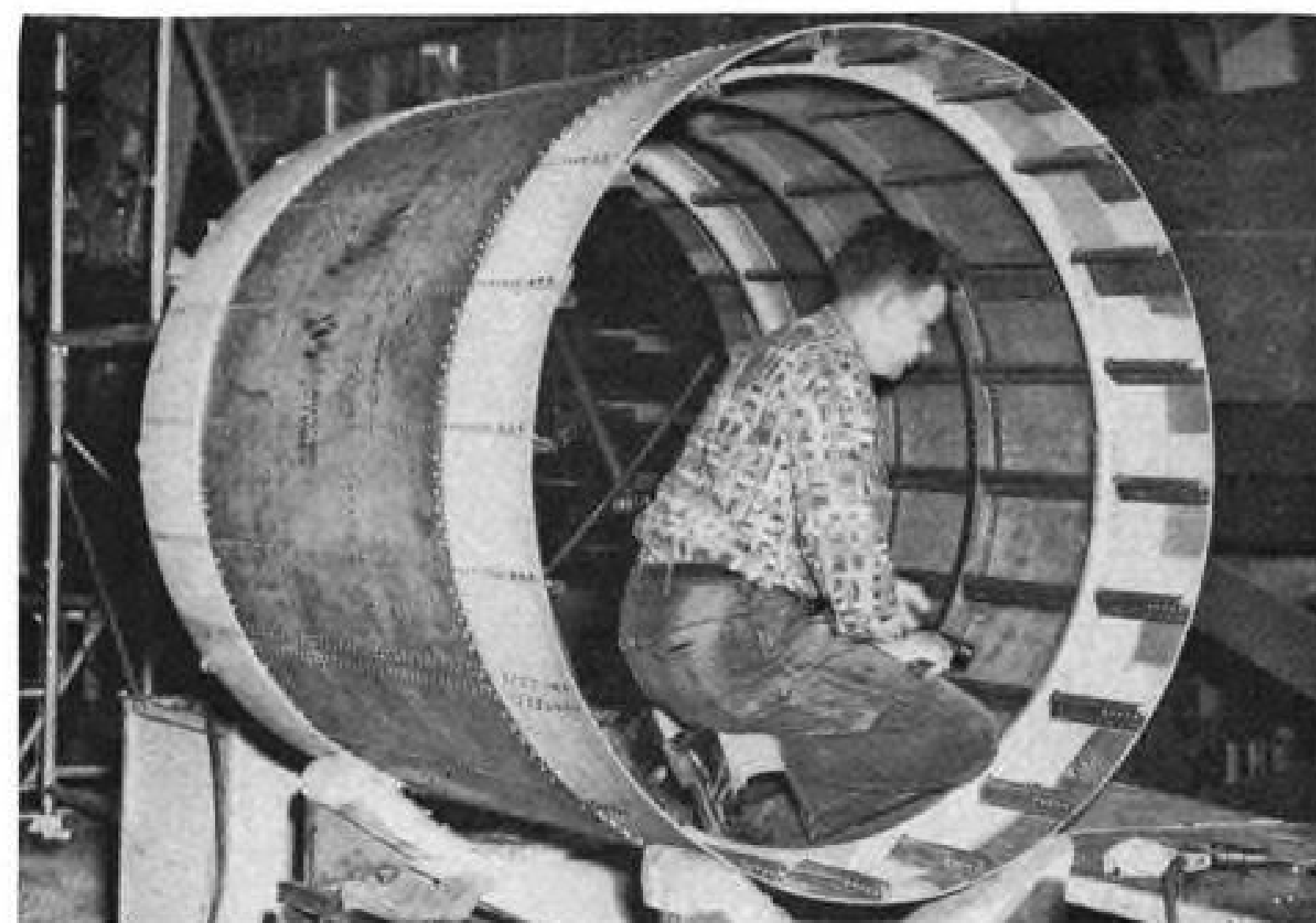
HORSION TEST CYLINDER in Republic Aviation's titanium studies has rolled skin (dark area), hot-formed channel formers and J-stringers.
