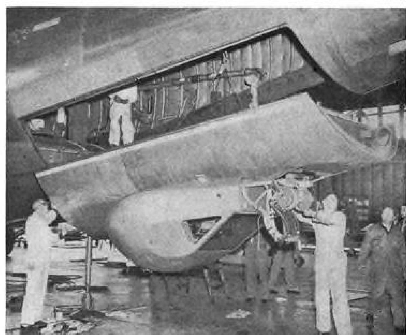
BOOM OPERATOR'S POD attaches to aft body.
