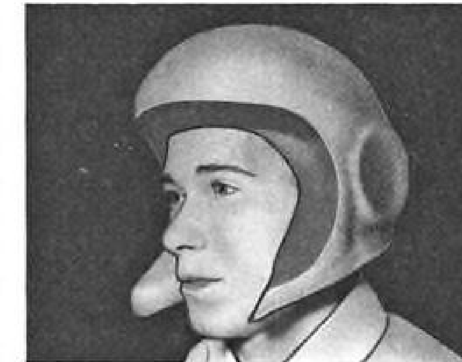
Flexible STAFOAM is here shown as helmet liner. Earpads of this material protect pilots against noise of jet engines. It is ideal as a packaging material.
