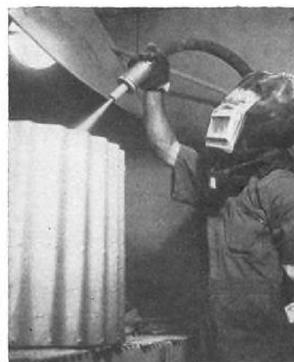
THIN-WALLED structures get high-temperature coatings without warping.
