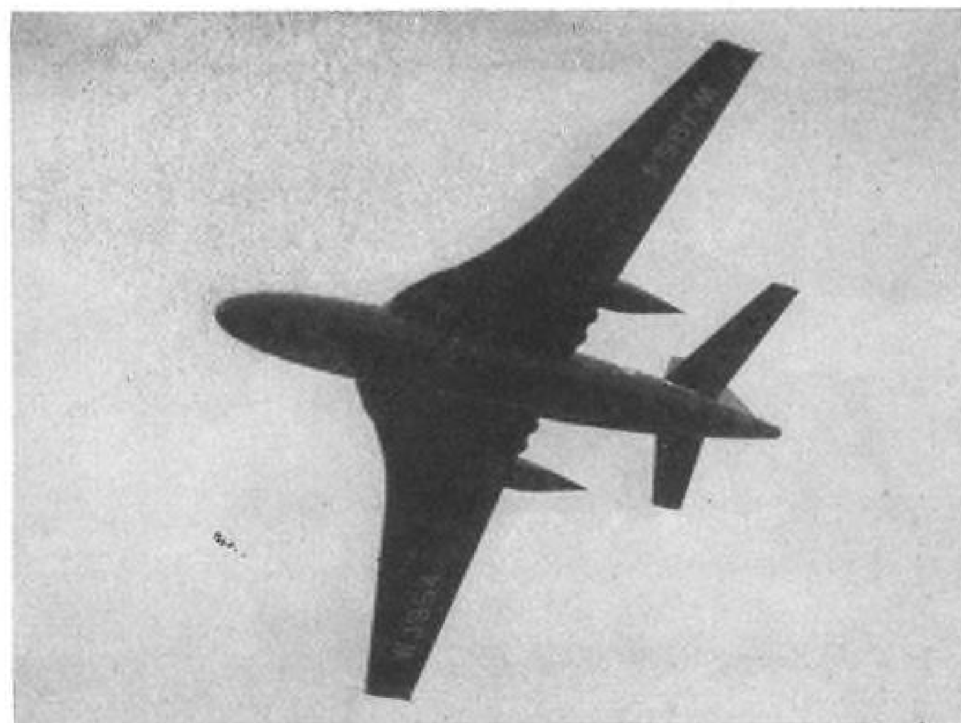
NACELLES for new rearward retracting landing gear trail behind wings of Vickers Valiant model B-2 bomber. Wheels folded outwards on prototype.
