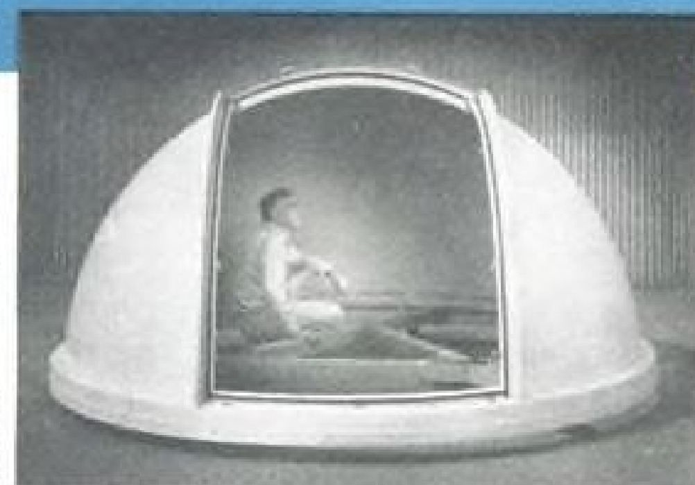
Dome open, showing smooth inner surface insulated both thermally and acoustically.
