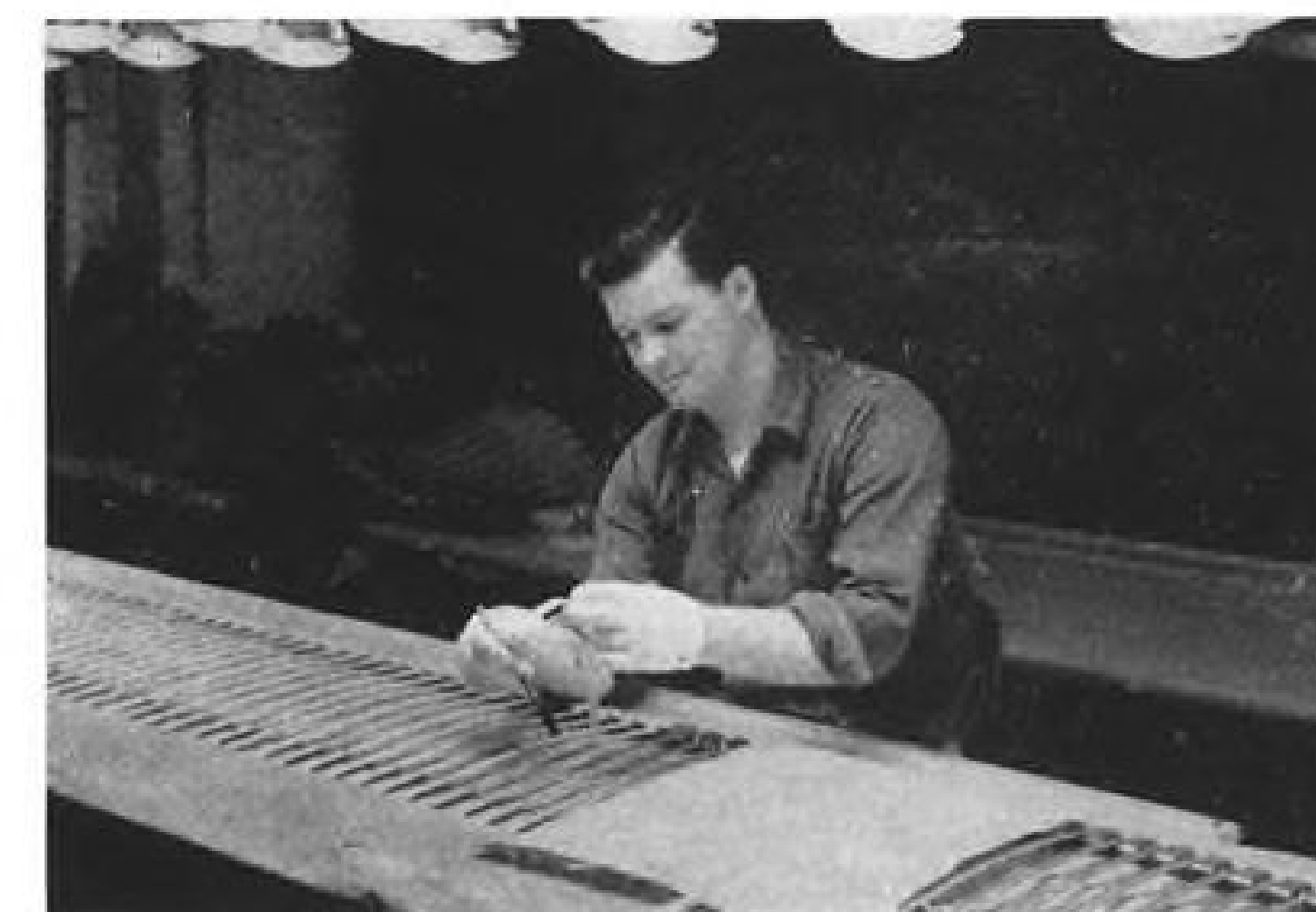
GLUING impregnated glass-cloth tape to corrugated aluminum alloy stiffener replaces hand application of many adhesive coats.
