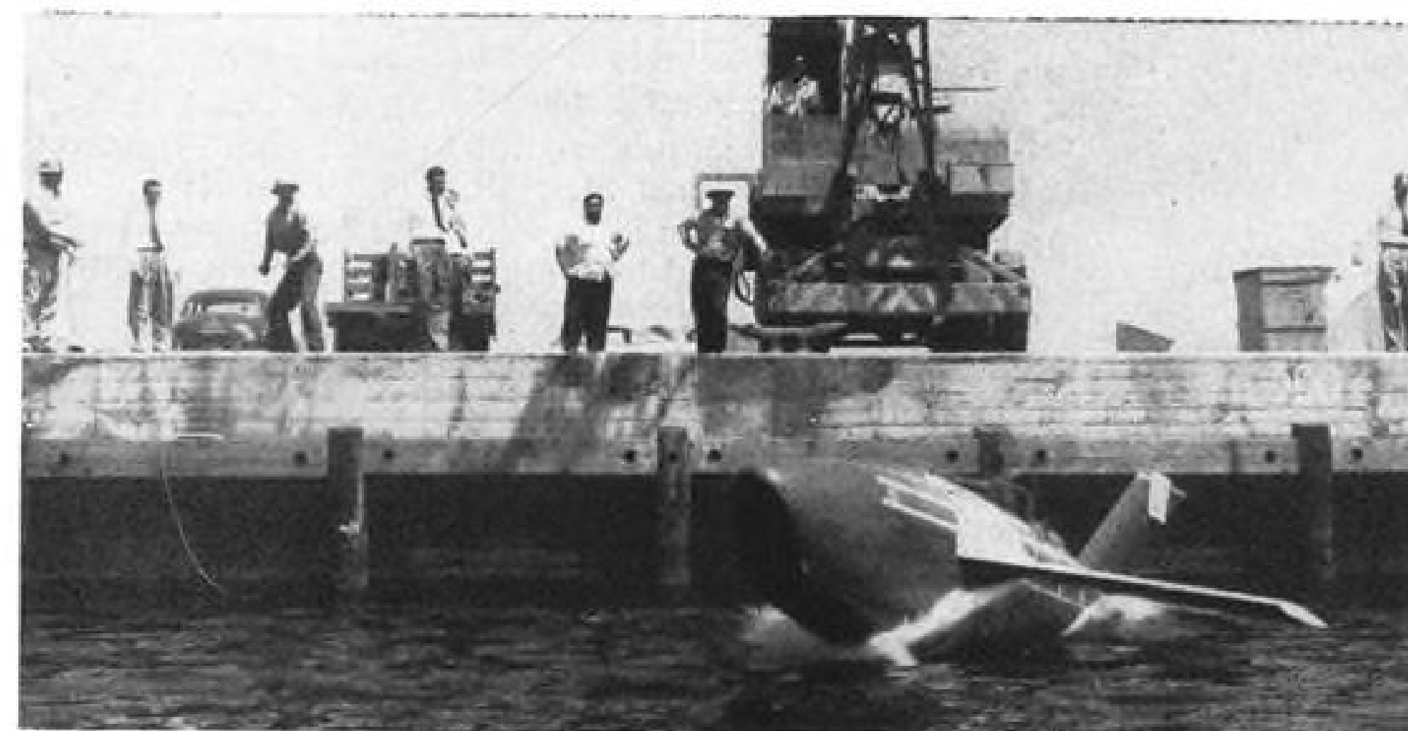
INTO THE WATER goes a Ryan XQ-2 at 20-ft./sec. rate to test flotation capability.
