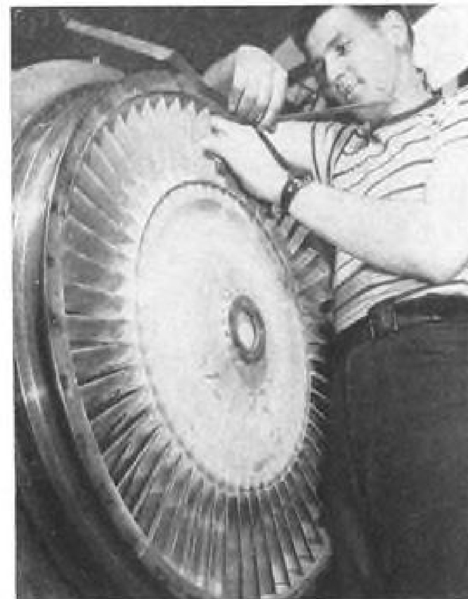
WASPALOY turbine blades have boosted thrust of P&WA J48 engine.
