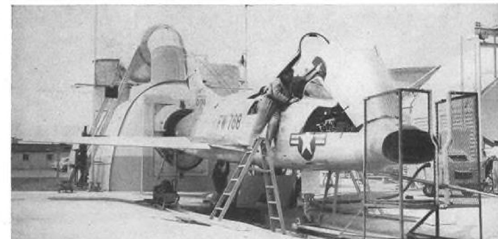
NORTH AMERICAN F-100 tailpipe fits in silencer unit during preflight check.
