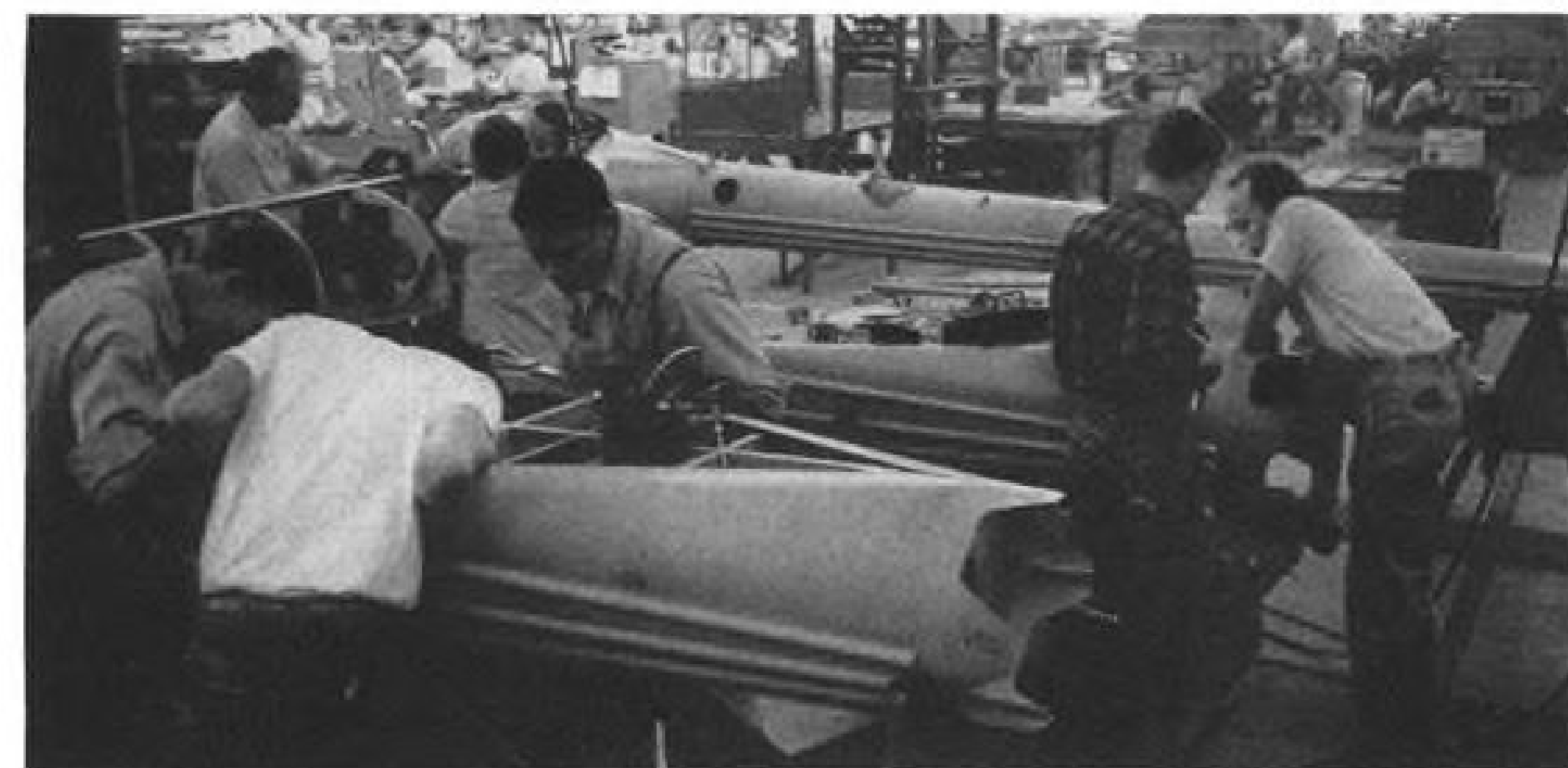
TAIL BOOMS for H-23s are fabricated on assembly line in Hiller's helicopter plant.
