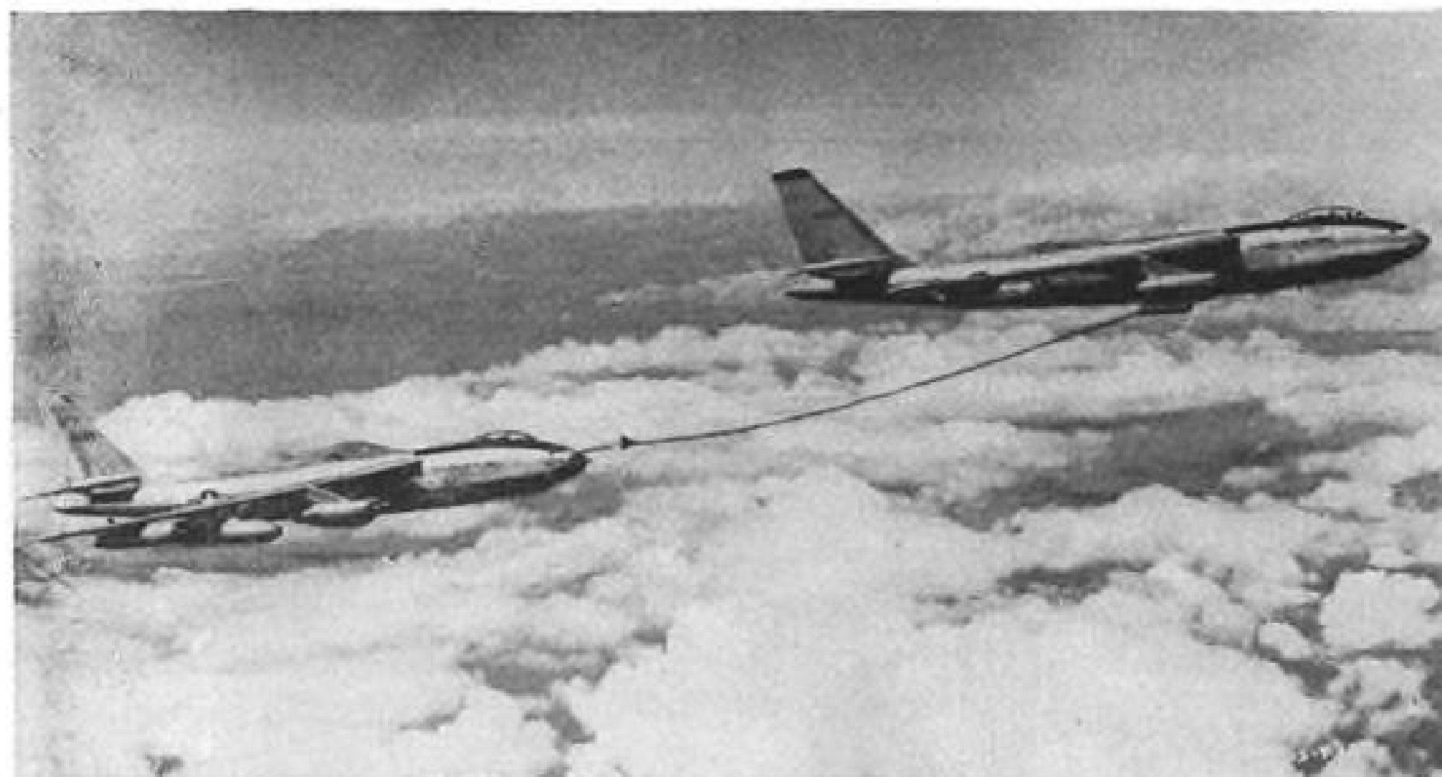
STRATOJET FEEDS STRATOJET—KB-47 (right) refuels B-47 via probe and drogue.
