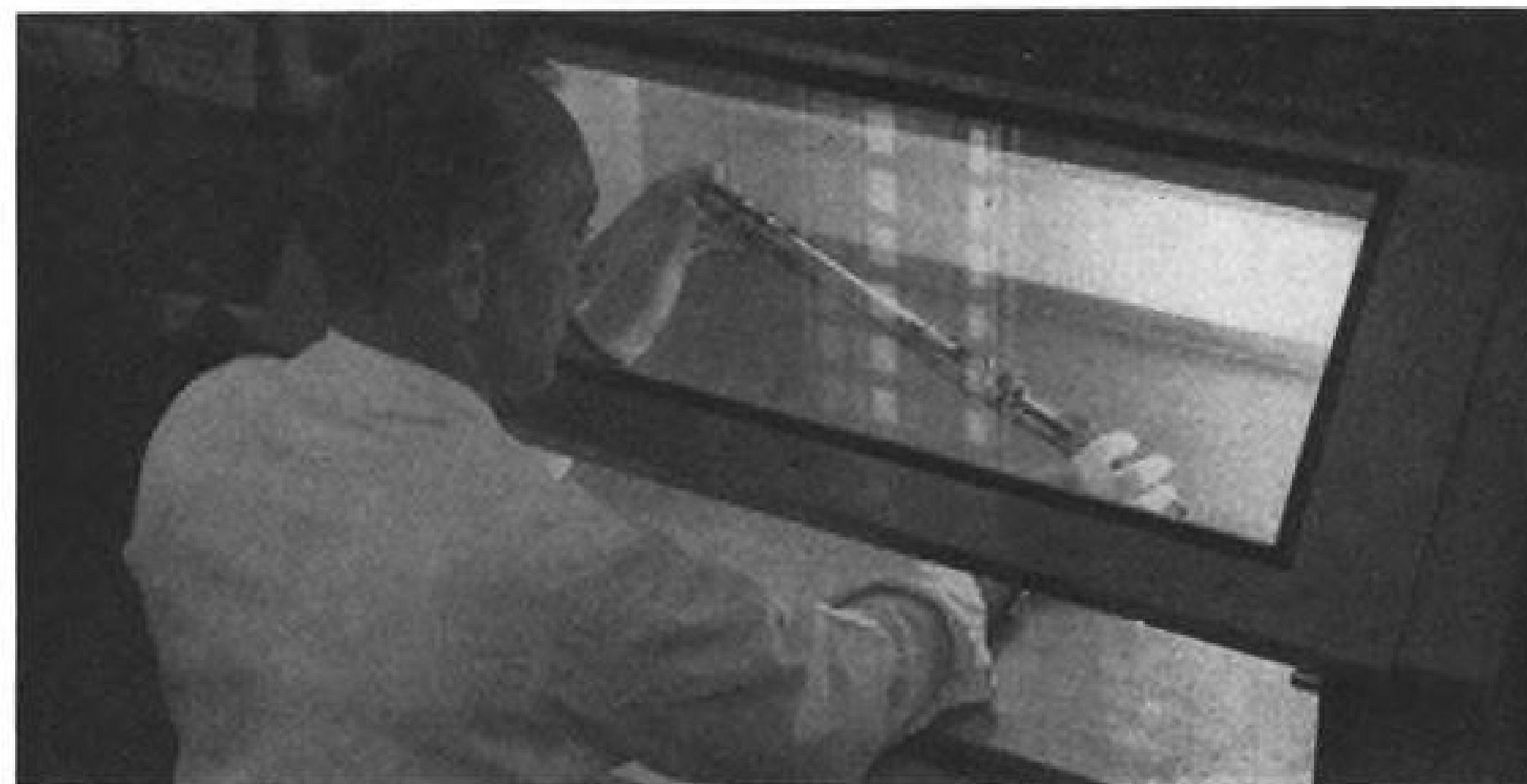
ELECTRONIC GUN is assembled under glass hood by technician wearing lint-free gloves.
