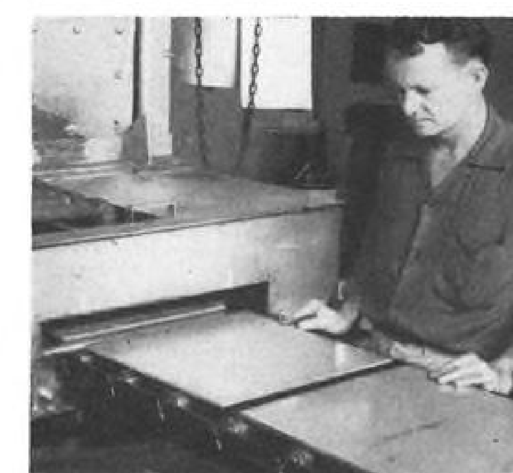
3. SANDWICHES get hot rolling, which fuses them; cold rolling lengthens them.
