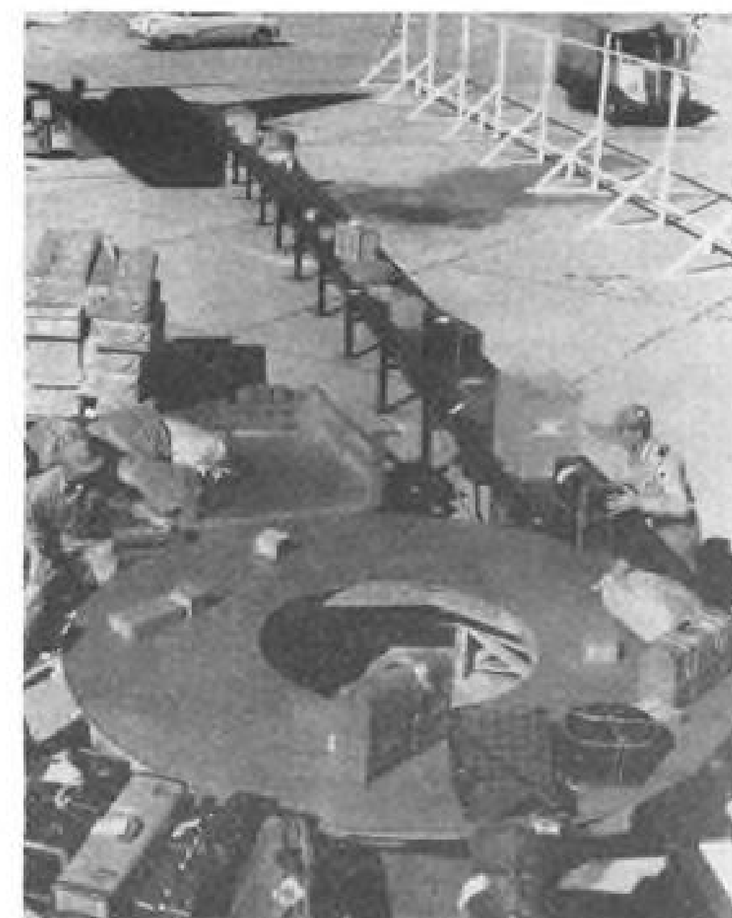
BAGGAGE movement is tested on working mockup of reversible conveyor at Denver.
