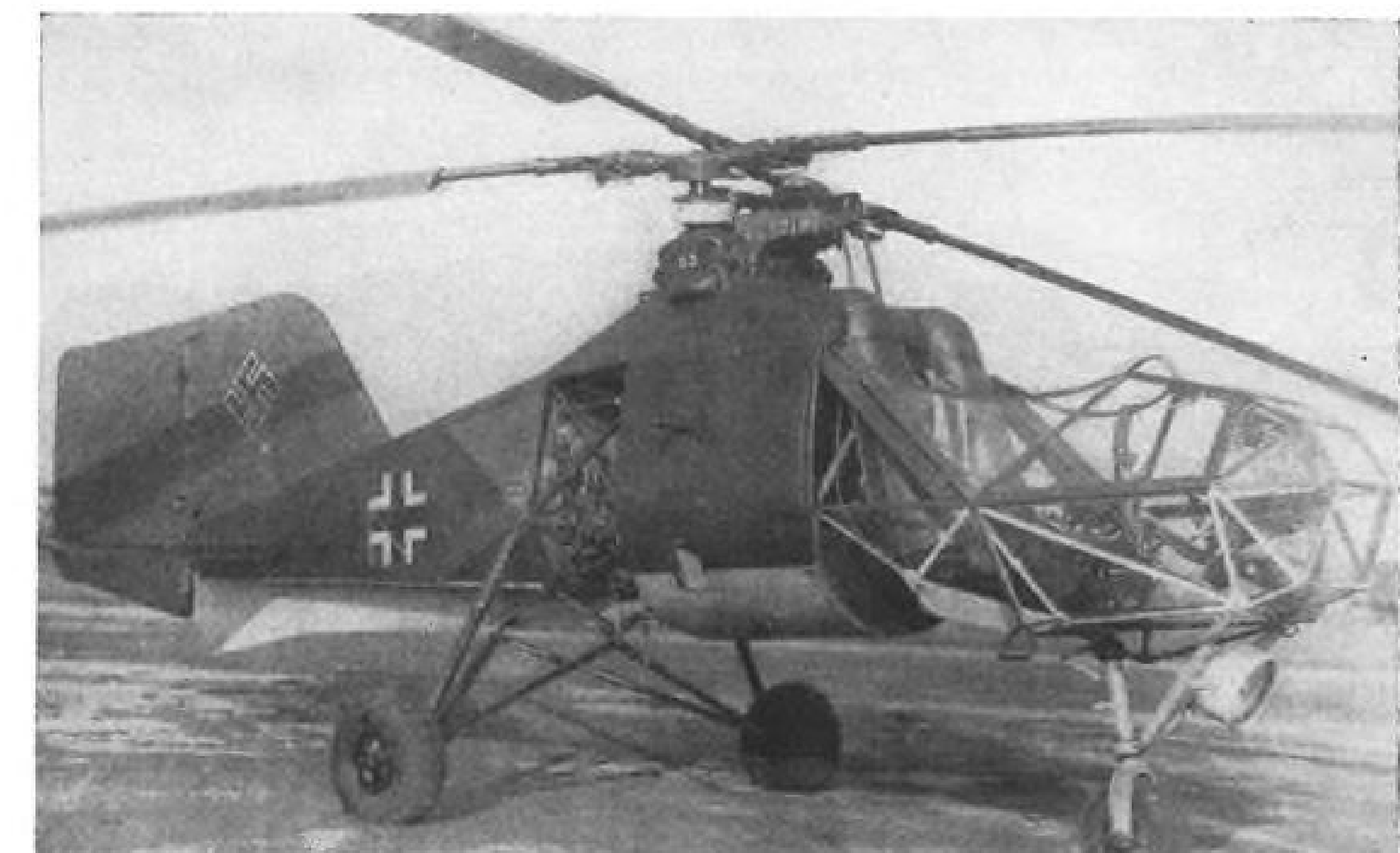
FL-282 HELICOPTER: Production version shown here was mainstay of German copter force in World War II; craft was built in 24 different models.
