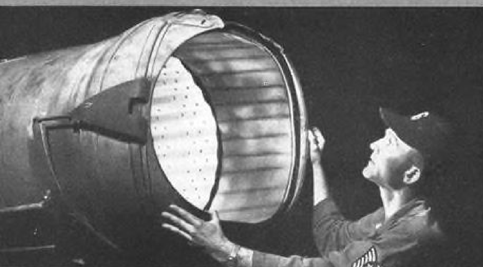
NEW, LARGER "EYELID" handles increased J47-GE-33 air-flow. Just inside 'lid, a sturdy ceramic-coated liner acts as a radiation shield, allows higher afterburner fuel flow; also preserves boundary layer cooling of the tailpipe.
