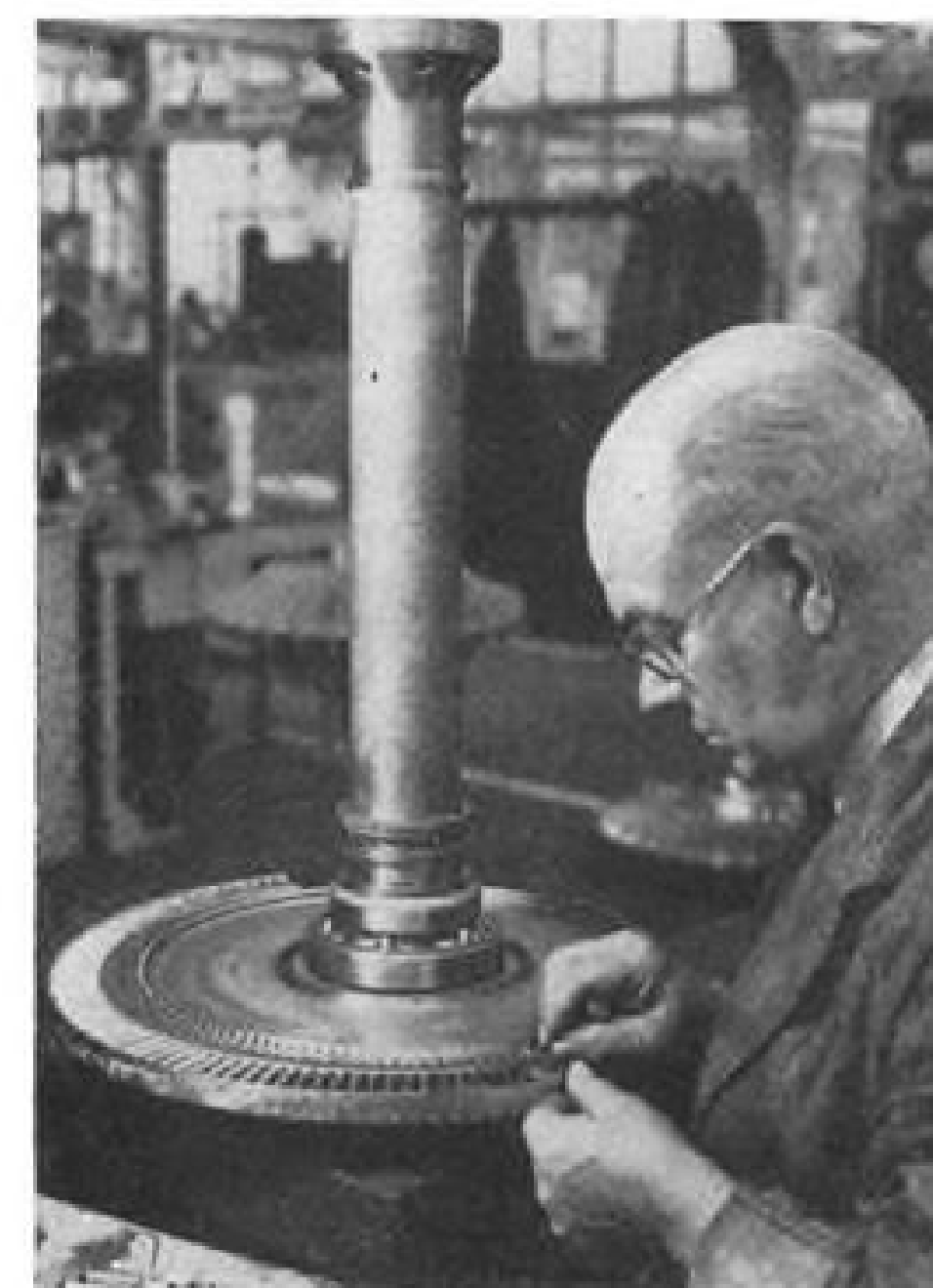
ROLLS-ROYCE TECHNICIAN fits shrouded turbine blades on Dart turbine.
