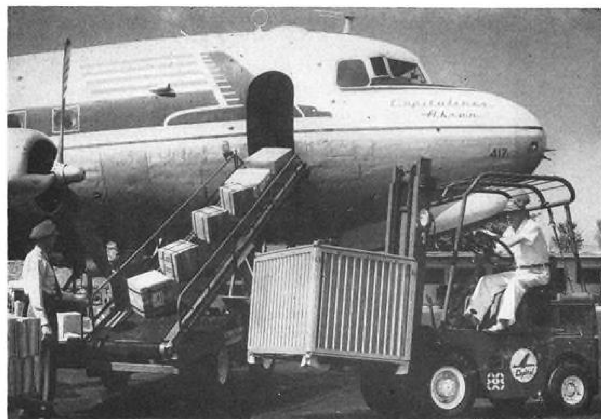
ALUMINUM PALLET for airfreight can be picked up by any of four sides by fork-lift.
